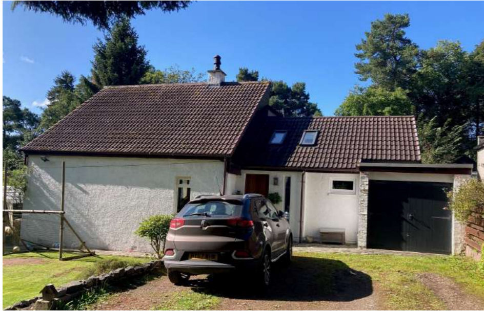
View of existing house from The Loan to the north east
