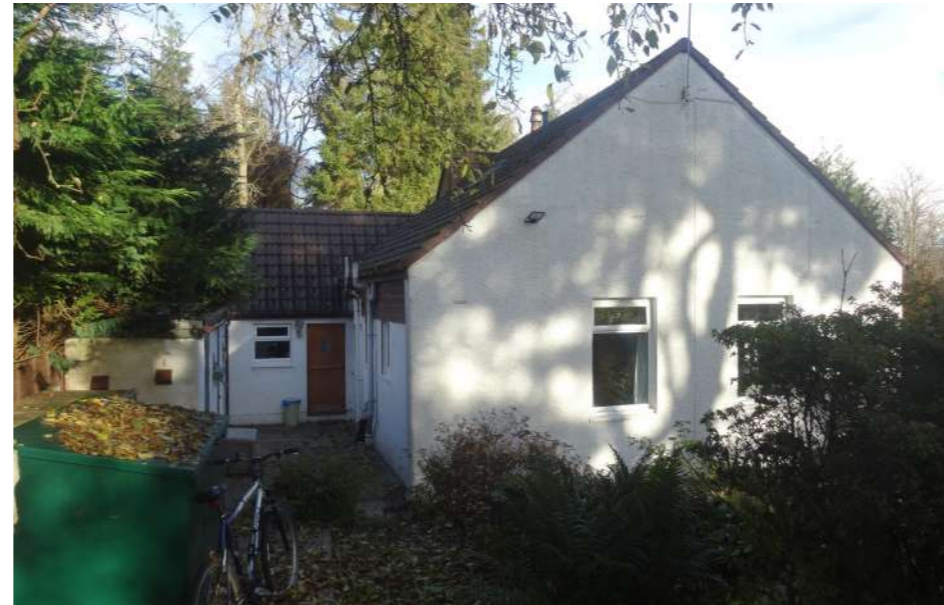
View of existing house from the south west
