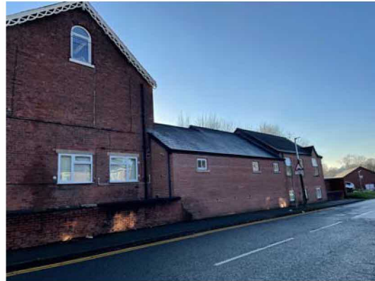
Photograph 6 – Existing North Elevation
