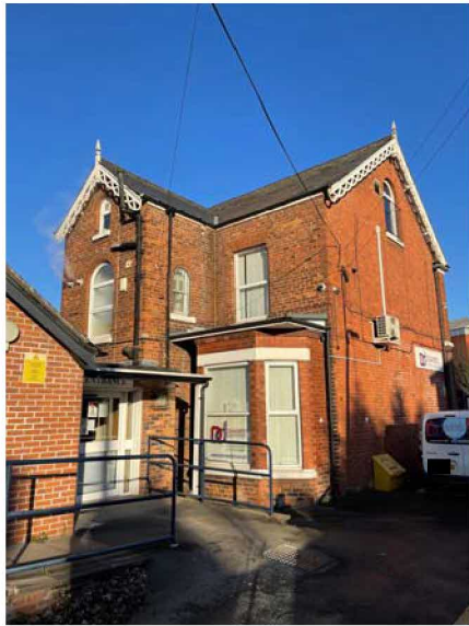
Photograph 4 – Existing West Elevation
