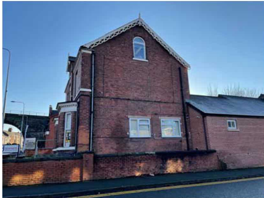
Photograph 5 – Existing North Elevation
