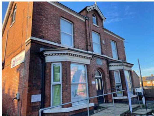
Photograph 1 – Existing East Elevation
