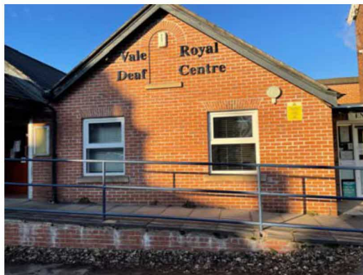
Photograph 3 – Existing South Elevation
