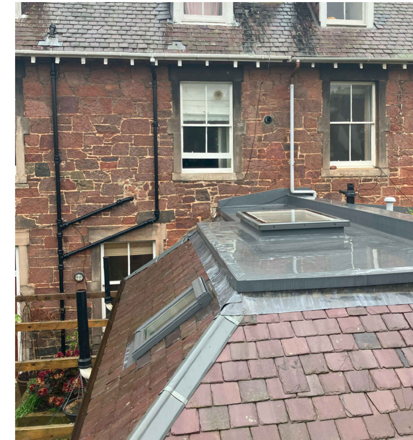
Site photo showing flat roof window and Velux roof window.
