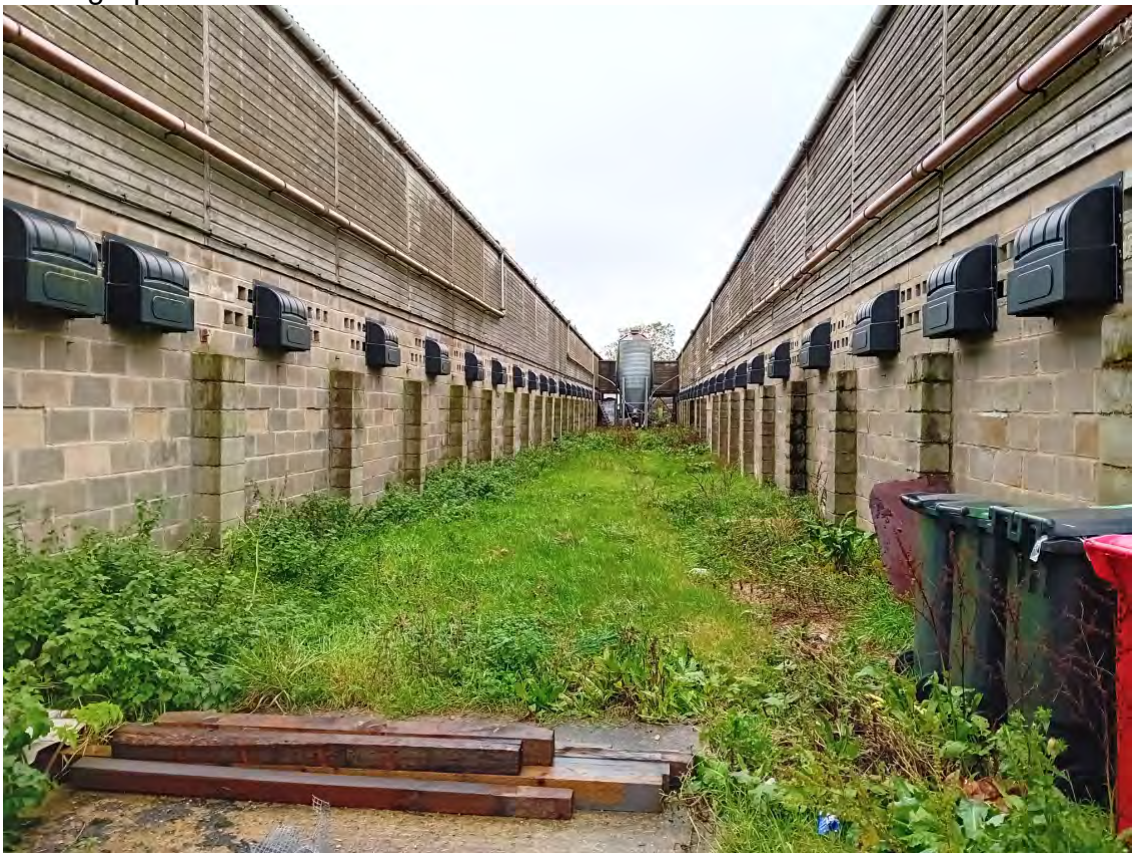
Photograph 14: Land between the two sheds.
