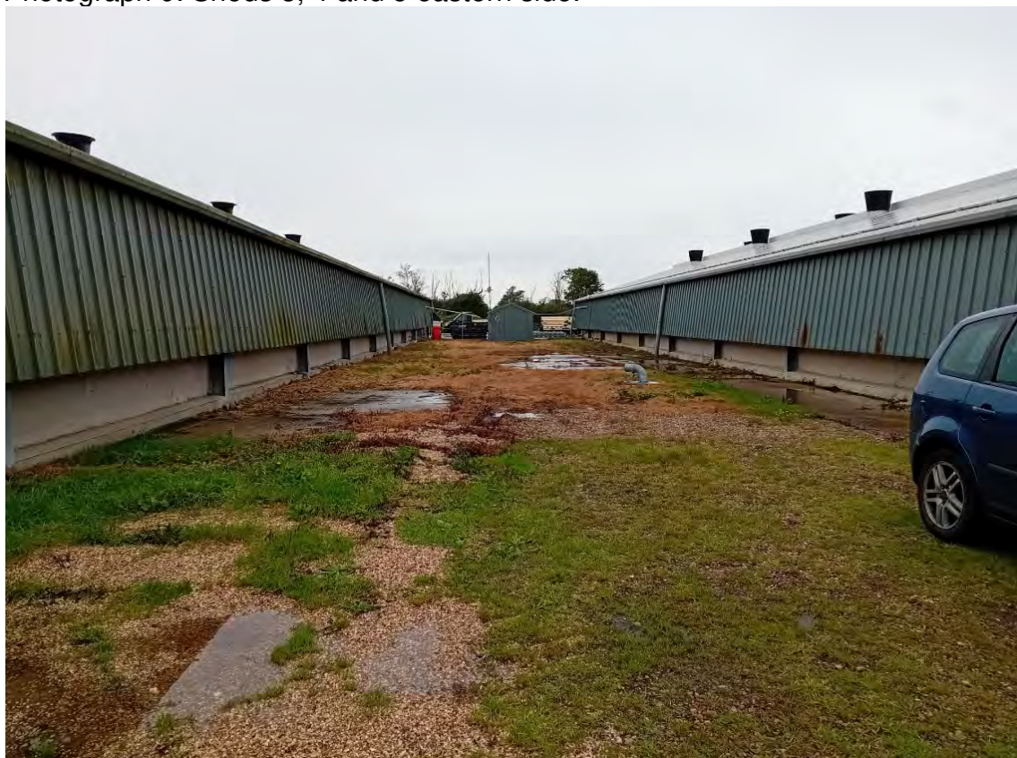
Photograph 10 : Land between shed 3 and 4 with below ground slurry tank
