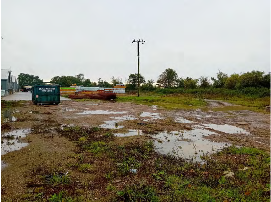
Photograph 3 : West side northern end. (new building location)
