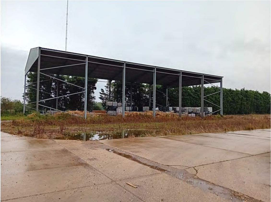
Photograph 21: Hay barn in the north eastern corner storing timber off cuts.
