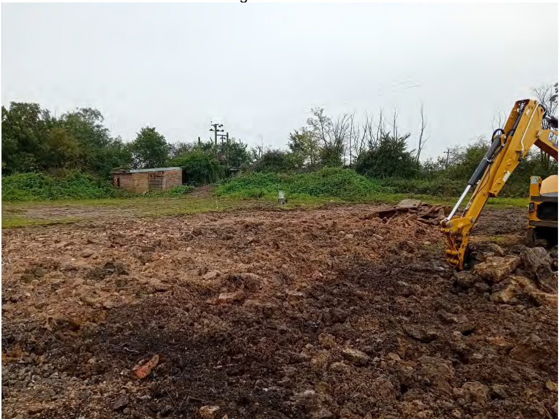
Photograph 2 : West side southern end. (new building location)
