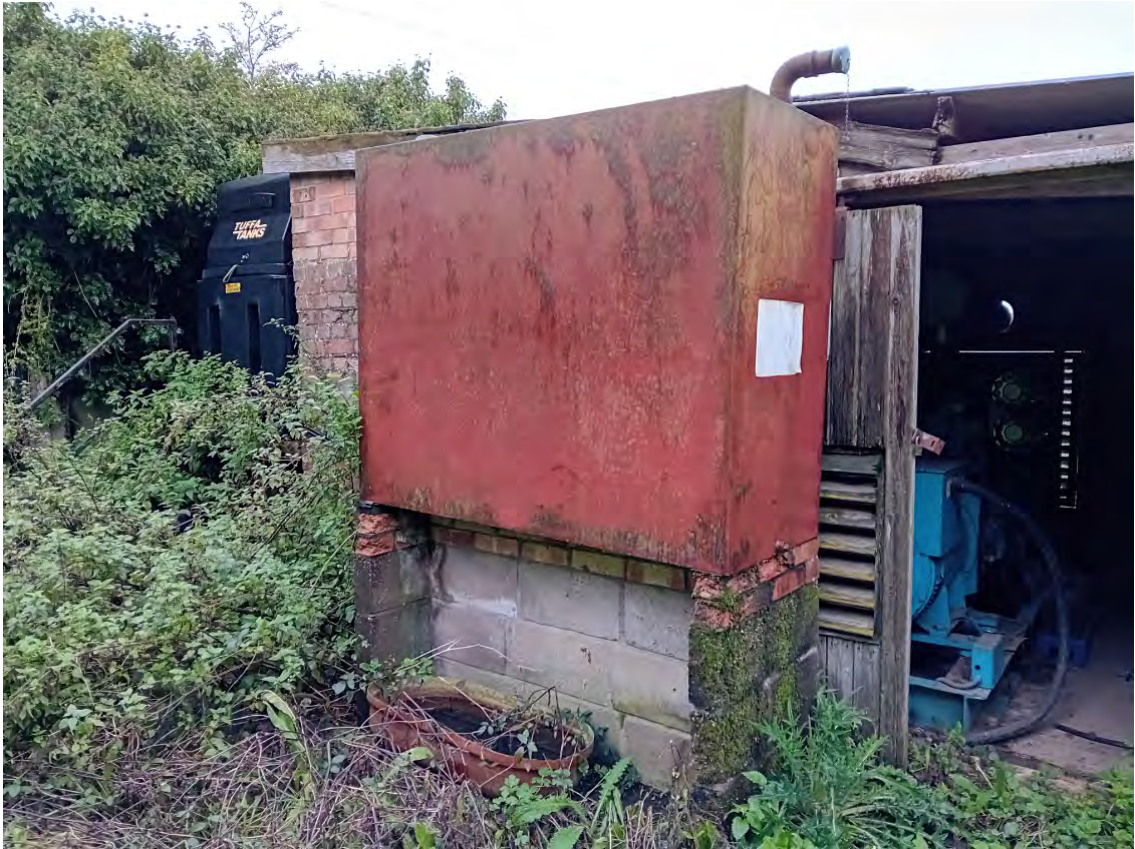
Photograph 5: Redundant tank to the rear of generator building
