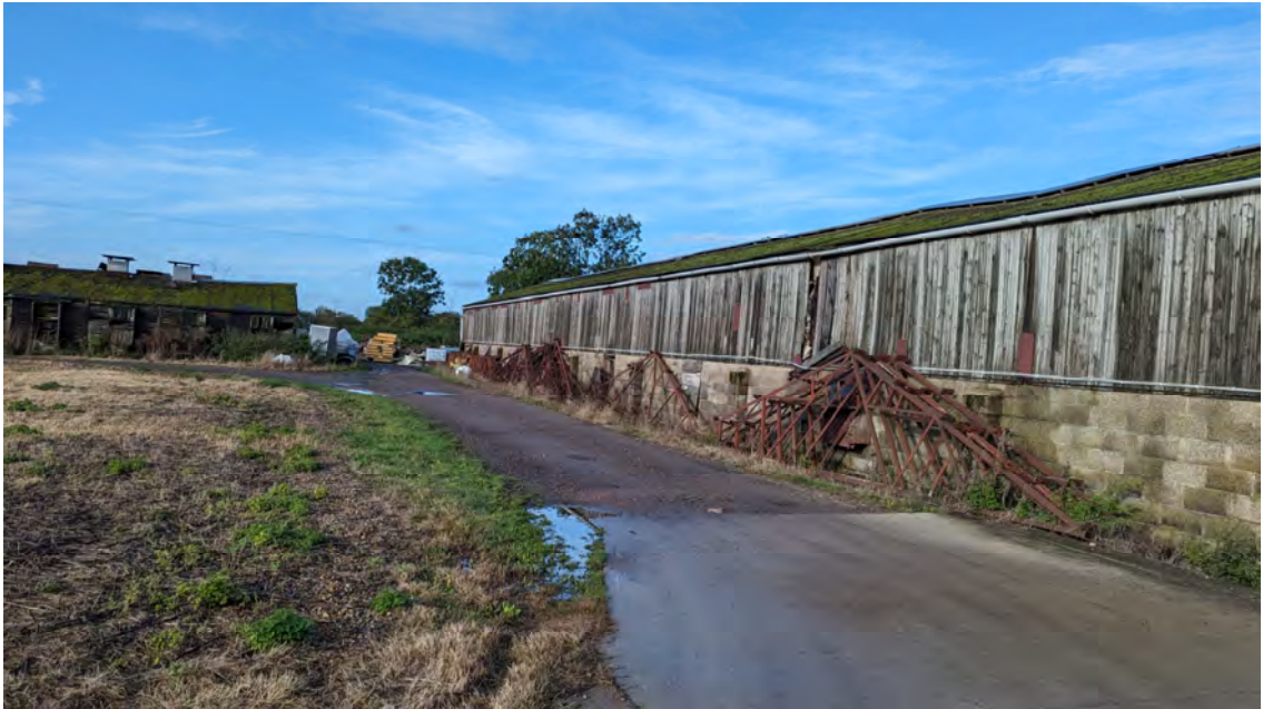
Photograph 19 : Shed 8 close to northern boundary.
