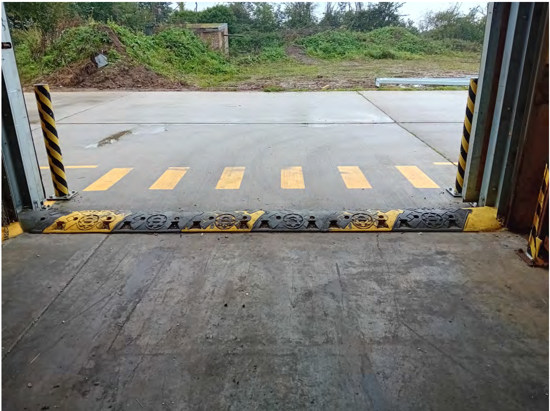
Photograph 7: Shed 3, hump installed for spill retention
