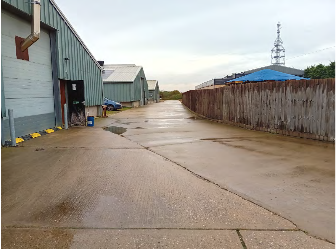
Photograph 9: Sheds 3, 4 and 5 eastern side.
