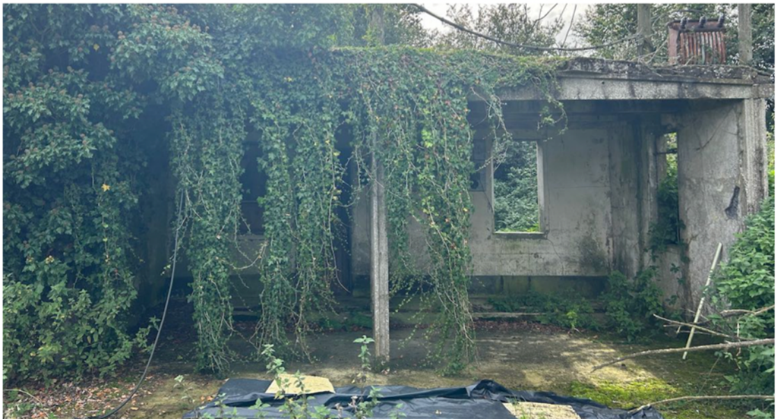
Photograph 1. Open sided structure
