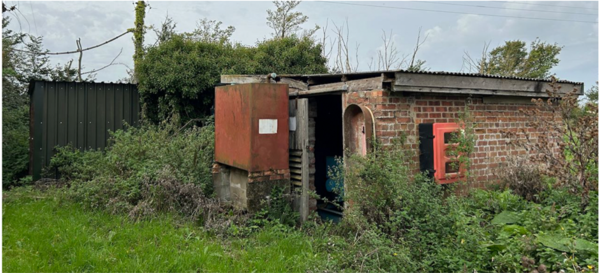
Photograph 2. Metal sheet building (left) and red brick building (right)
