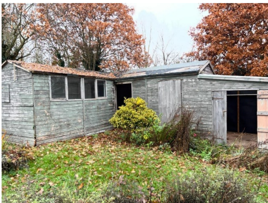
Figure 3. Outbuildings/Office & Sheds (Recently removed)
