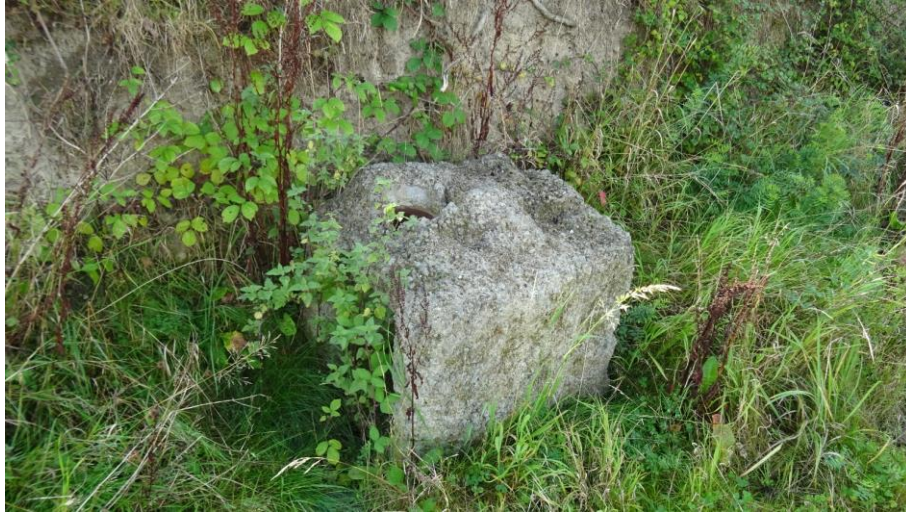
Figure 2.2. Concrete to be removed with the assistance of a machine
