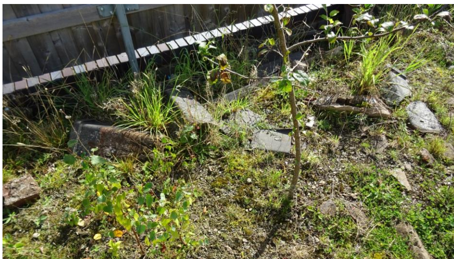
Figure 2.1. Rubble and roof tiles to be removed by hand
