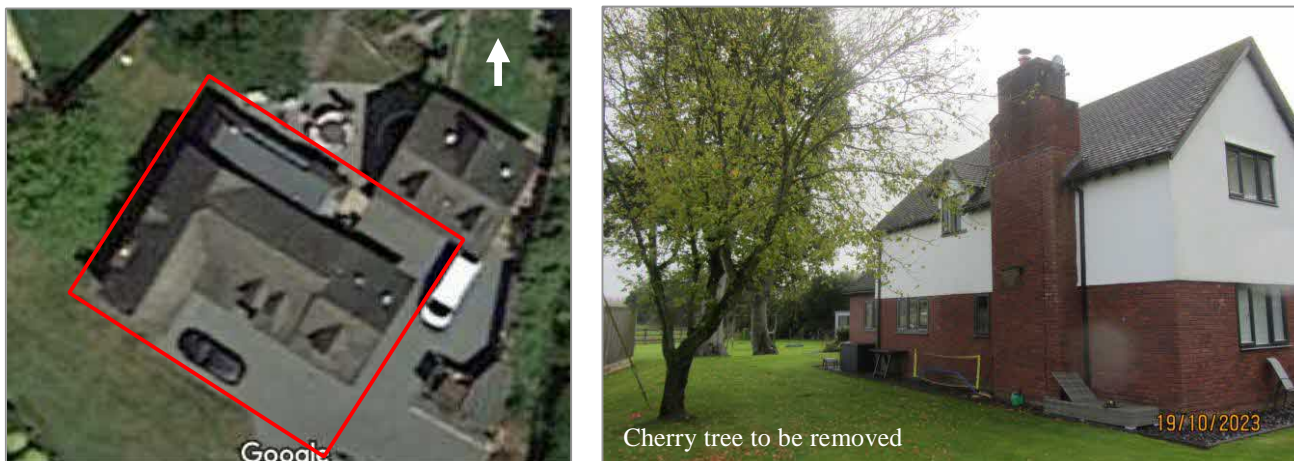
Fig.1. Application building (Google). Fig.2. Northwest elevation and southwest gable.
