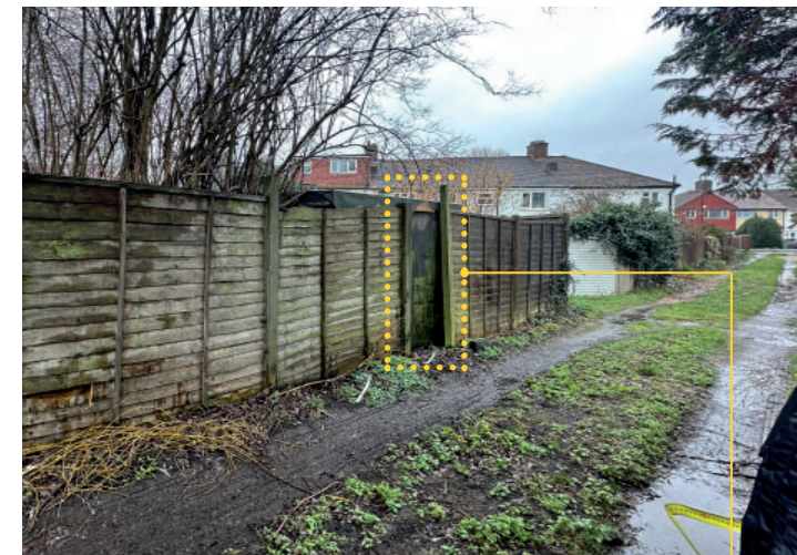
View of the rear garden fence from the Alleyway, indicates former access.
