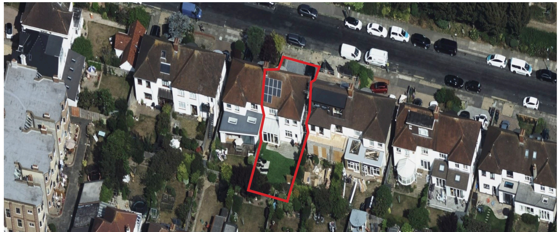
Figure 01.1: No. 44 Saxon Road front (top) and rear (bottom) bird's eye view
