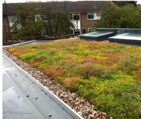
Sedum roof with roof light
