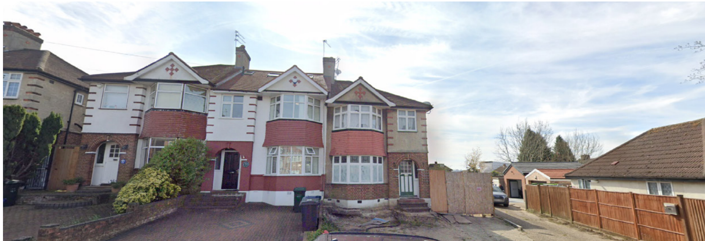
1. Street View of 141-145 Arlington Rd.
