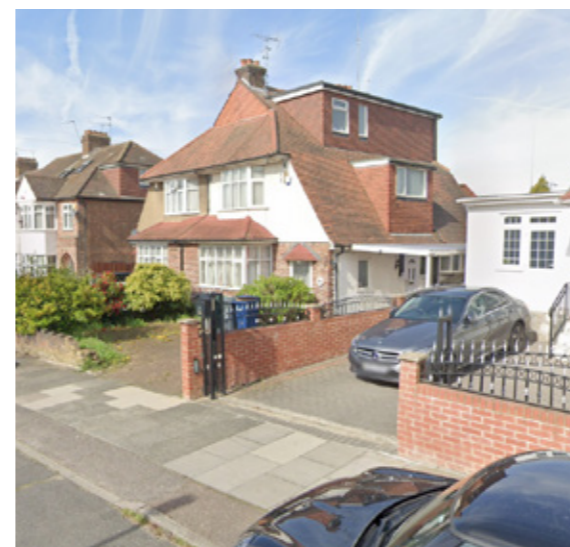
4. Street View of 94 Arlington Rd.
