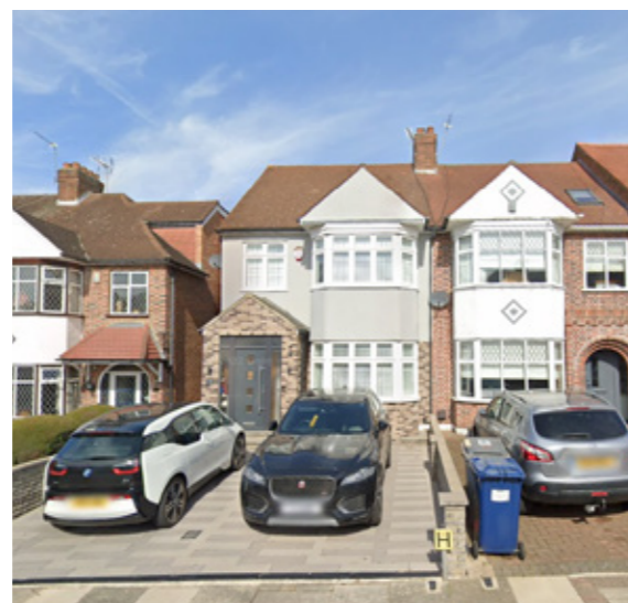
3. Street View of 110-114 Arlington Rd.
