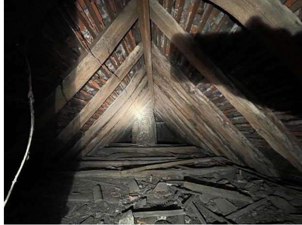
Photograph 8. The central section of the loft space.
