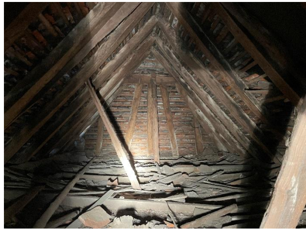
Photograph 10. The northern section of the loft space.
