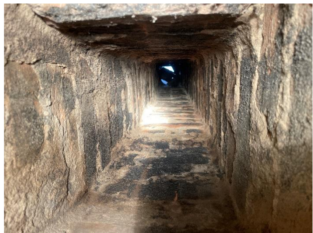
Photograph 6. The interior space within the southern chimney stack.
