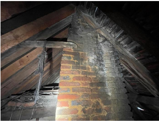
Photograph 9. The chimney stack within the central section of the loft.
