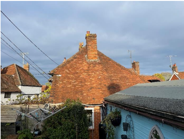
Photograph 3. The southern elevation of the building, showing the southern chimney stack.
