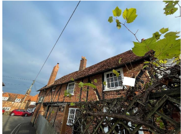
Photograph 2. The western elevation of the building.
