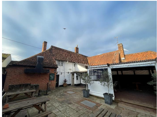
Photograph 4. The building viewed from the south-east.
