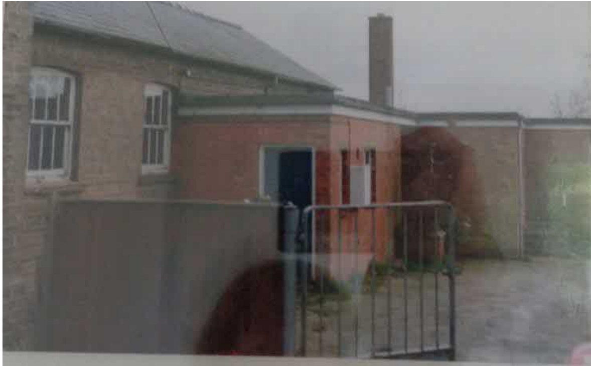
Photo c1991 showing the building pre-conversion (Applicants)
