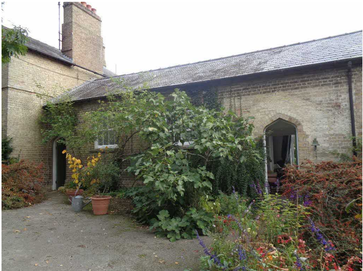
The rear of the former schoolhouse and school room looking east
