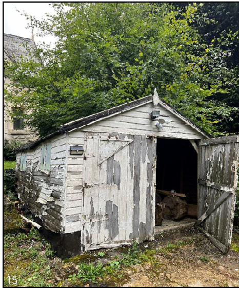
Plate 15. View of the garage from the north-east.
