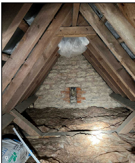
Plate 9. Internal view of Loft Void B
