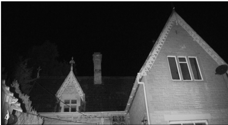
Plate 4. Field of view of the IR camera deployed on the eastern elevation (Survey Point 4).
