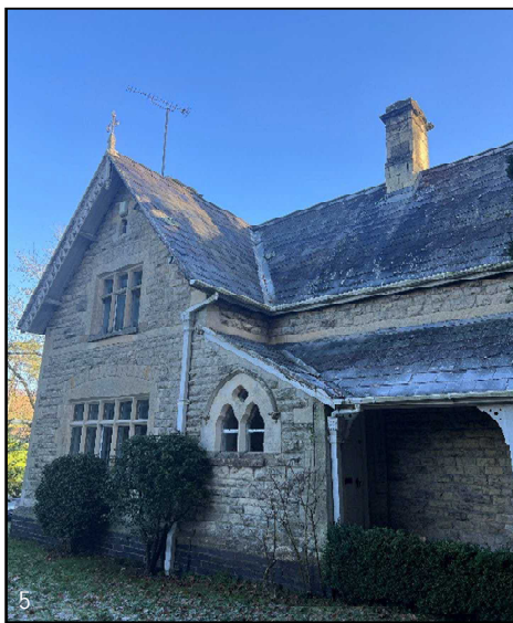
Plate 5. View of the building from the south-west
