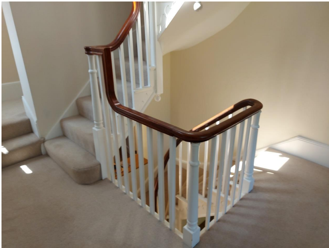
Figure 14: The stair at first floor level
