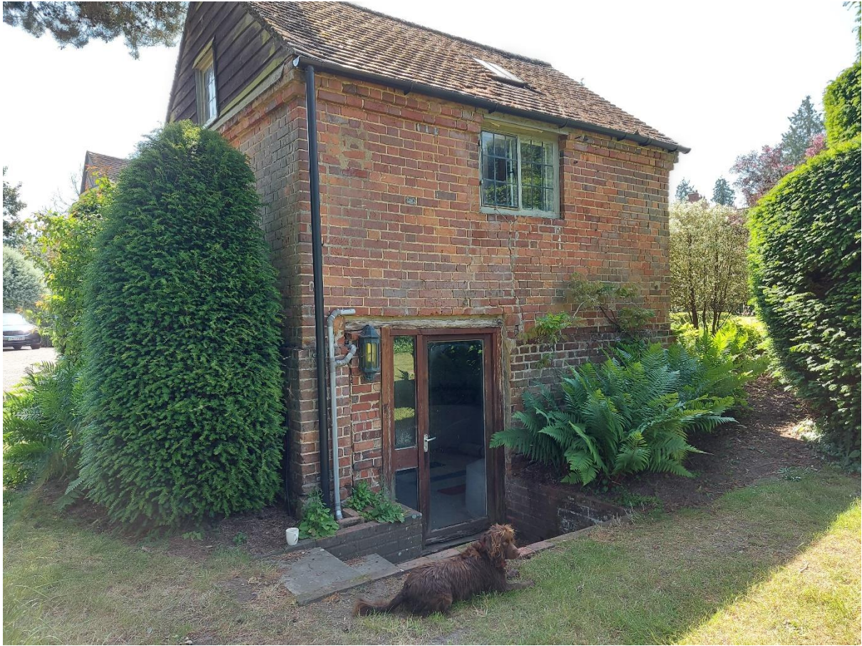
Figure 15: The west side of the granary to the west of the main house
