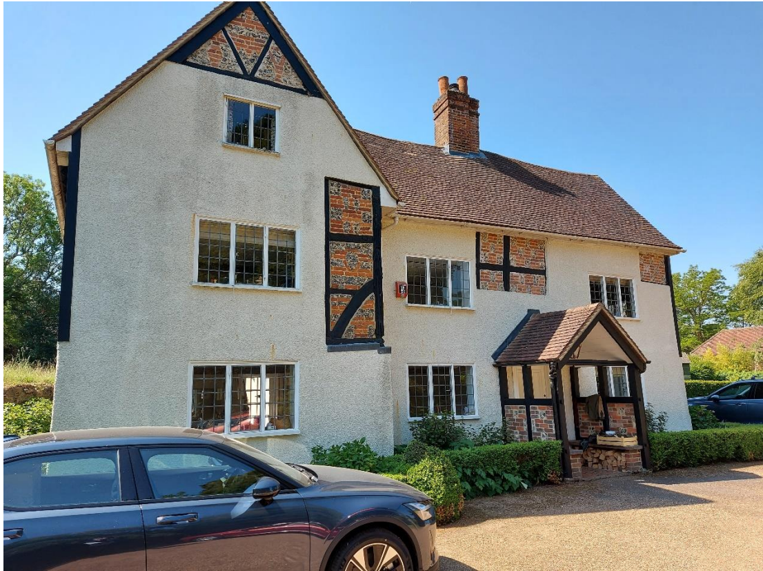
Figure 7: The main north-facing front
