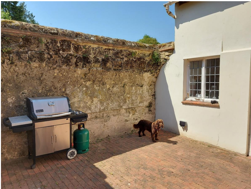
Figure 10: The remains of a stone vaulted space set into the bank Behind the house
