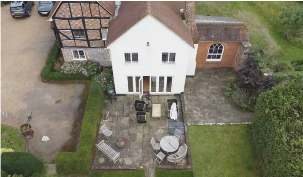
Overview from the west, with 1991 extension prominent
