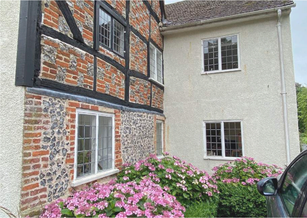
Juxtaposition of original house construction (left) and 1991 extension (right)
