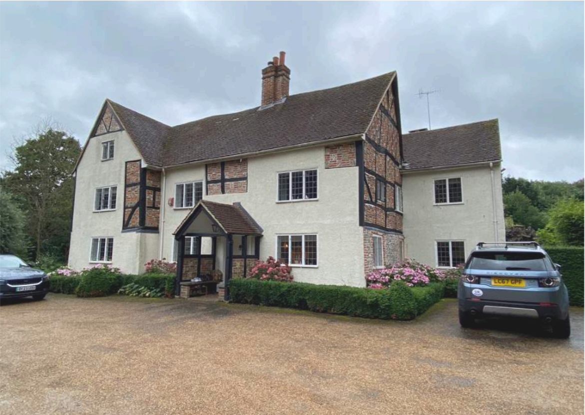
Primary facade of the house, northern elevation from the driveway
