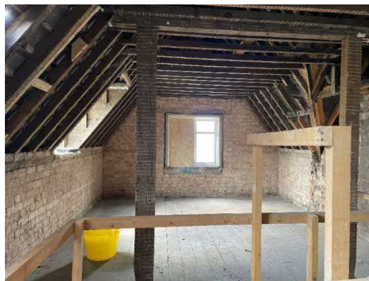
Plate 32: Second floor space in the southern part of the building.
