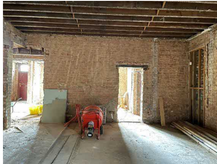
Plate 24: View west within the rear space on the ground floor.
