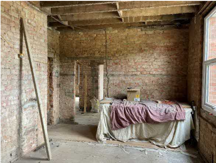
Plate 27: First floor space at the front of the property.
