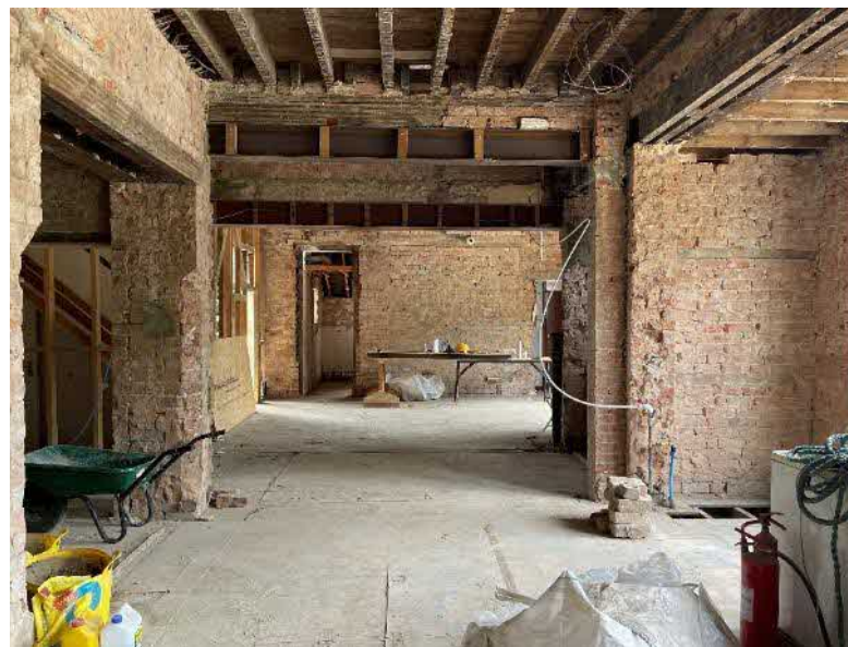
Plate 21 View south in front space on the ground floor.
