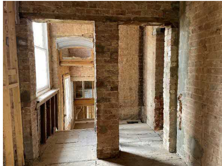
Plate 29: Detail of decorative arch and layout at first floor.
