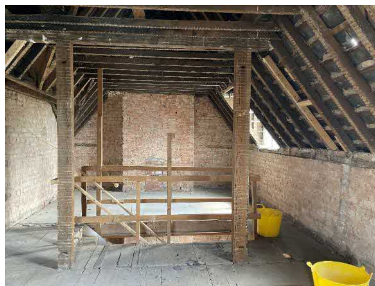
Plate 31 Second floor space in the southern part of the building.
