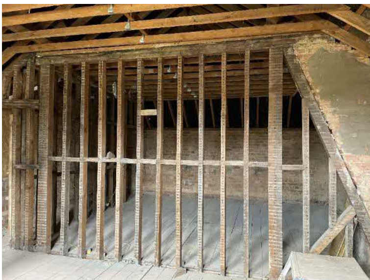
Plate 33: Second floor space in the rear of the building.
