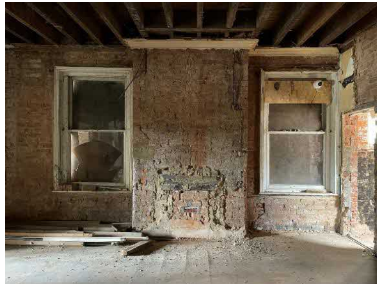
Plate 25: Detail of chimney breast, sash windows and window surrounds on the northeast elevation at ground floor.
