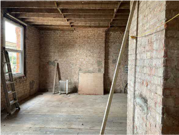
Plate 26: First floor space at the front of the property.
