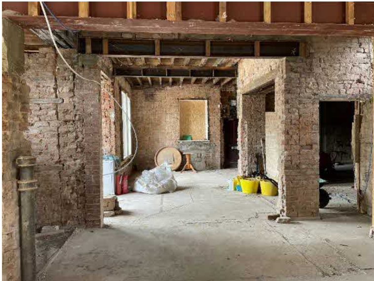
Plate 22: View north in front space on the ground floor.
