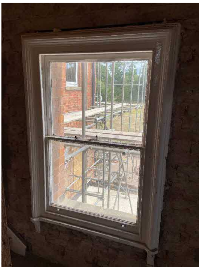
Plate 30: Detail of window surround on the first floor.
