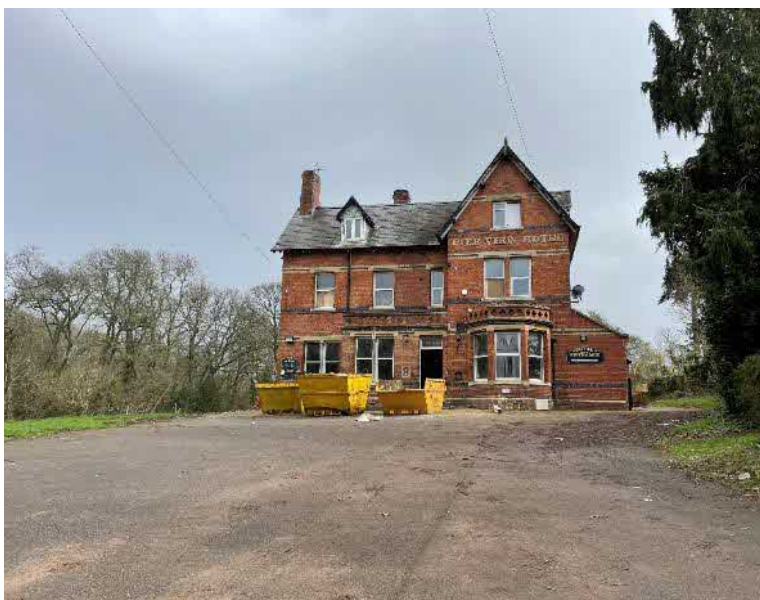
Plate 3: View east across the Site from Oldminster Road.
