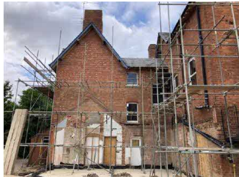
Plate 20: Areas adjacent to the southeast elevation as now extant.
