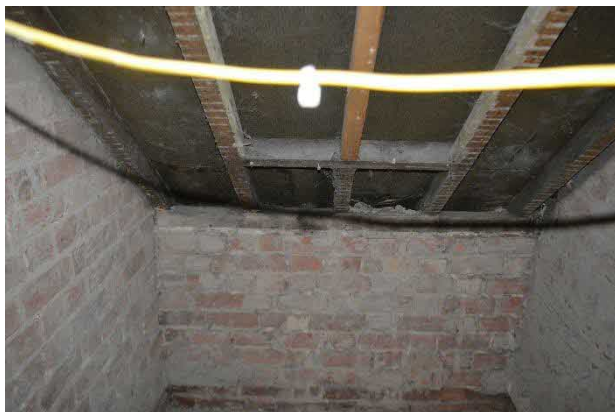
Photograph 24: Small room to the east of building
