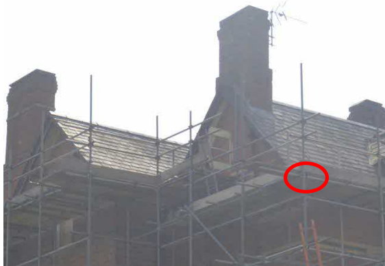
Photograph 5: Northern elevation gables and EM3 location
