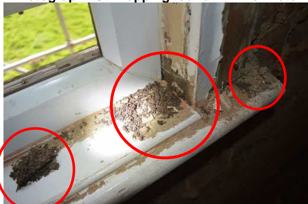
Photograph 20: 1000s of droppings found in top floor room beneath the NE gable
