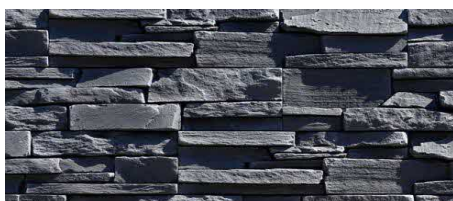
Stone detailing to rear decorative screen of covered area.
