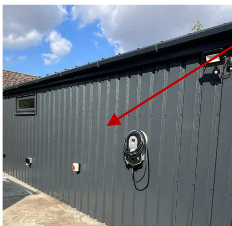
Rear & side elevations to have aluminium vertical cladding.
