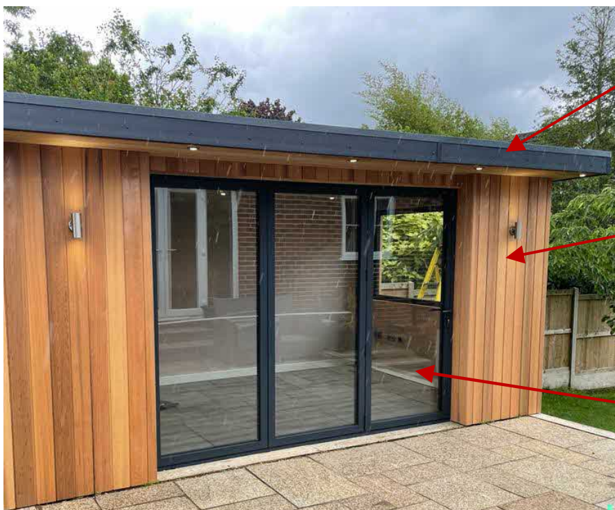
Rear & side elevations to have aluminium vertical cladding.
