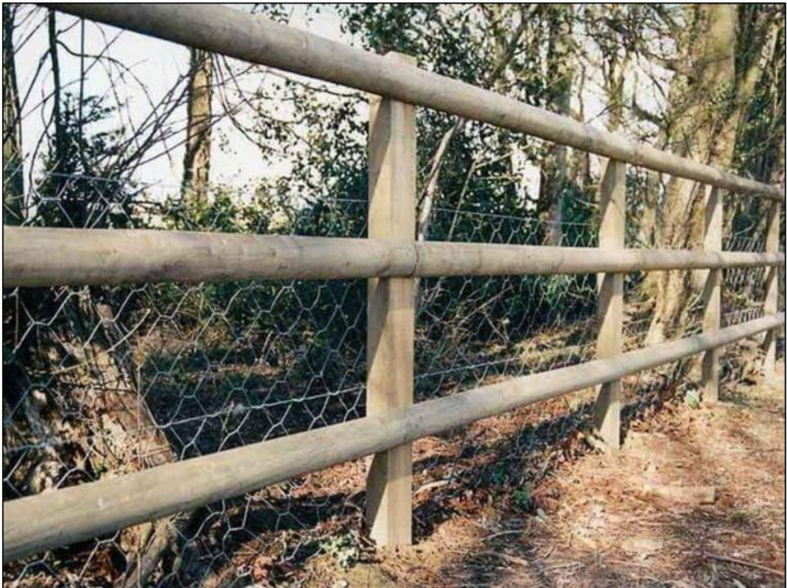
Figure 2: Nailed square post and rail fencing with low level galvanised wire netting.
