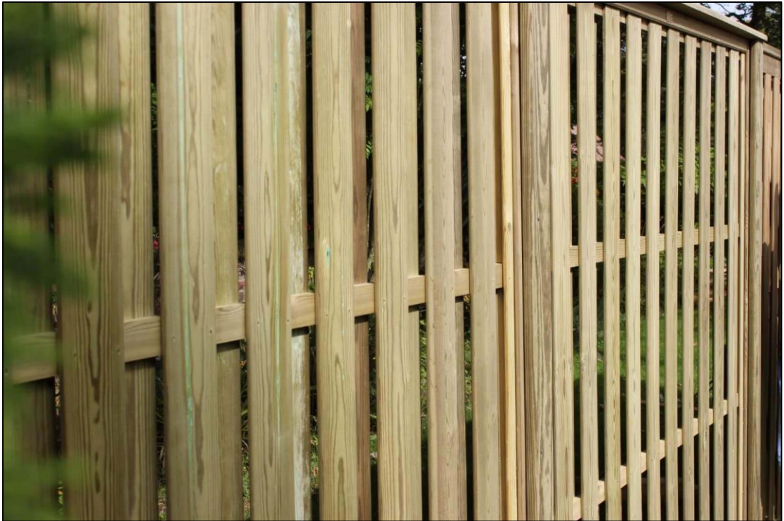
Figure 1: Hit-and-miss natural timber fencing.
