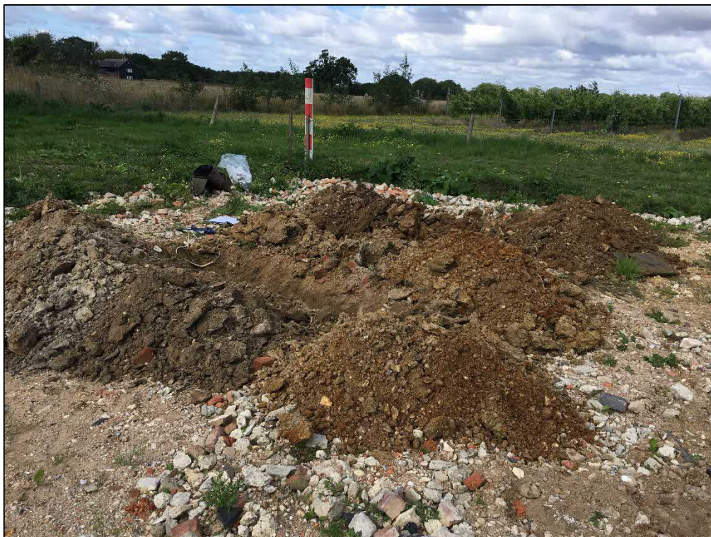
Photograph 7: Location of TP2 and TP3.
