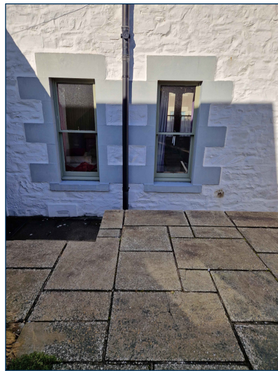
Photo of Original South Elevation Windows
