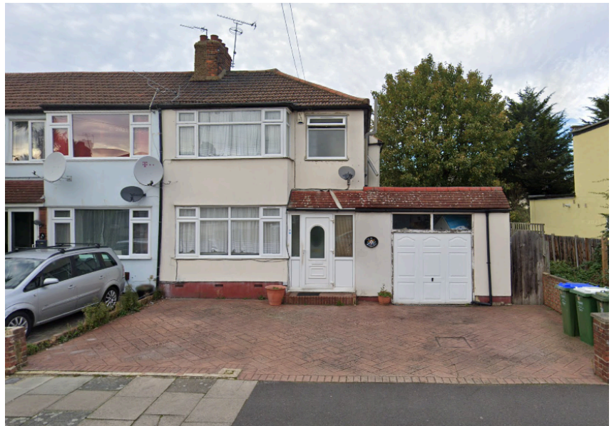
Image 2 – Existing north looking view onto the application site.
