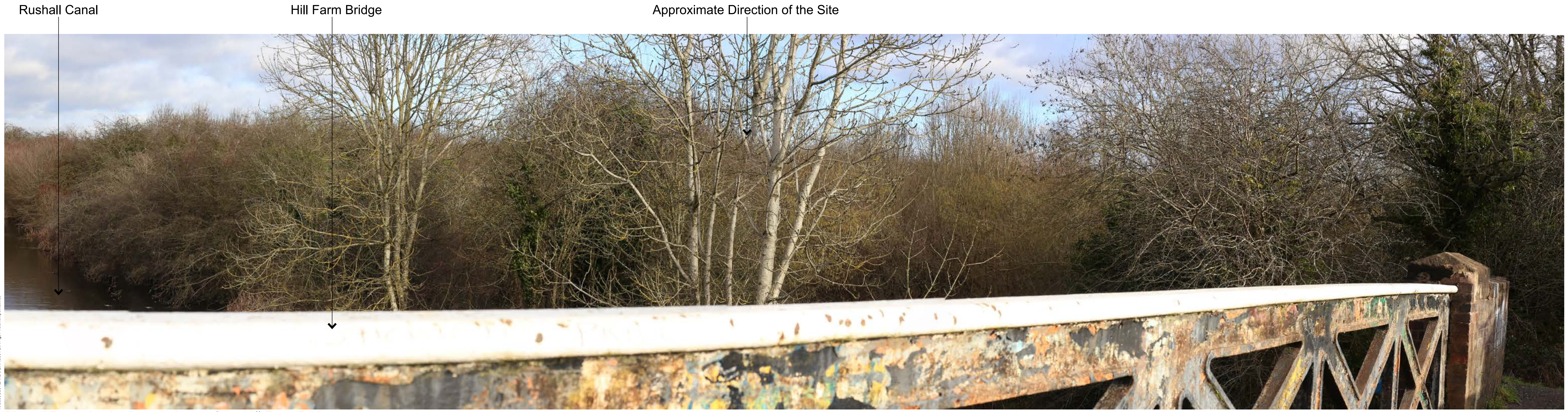
Photo Viewpoint 6: View north-east from Hill Farm Bridge
