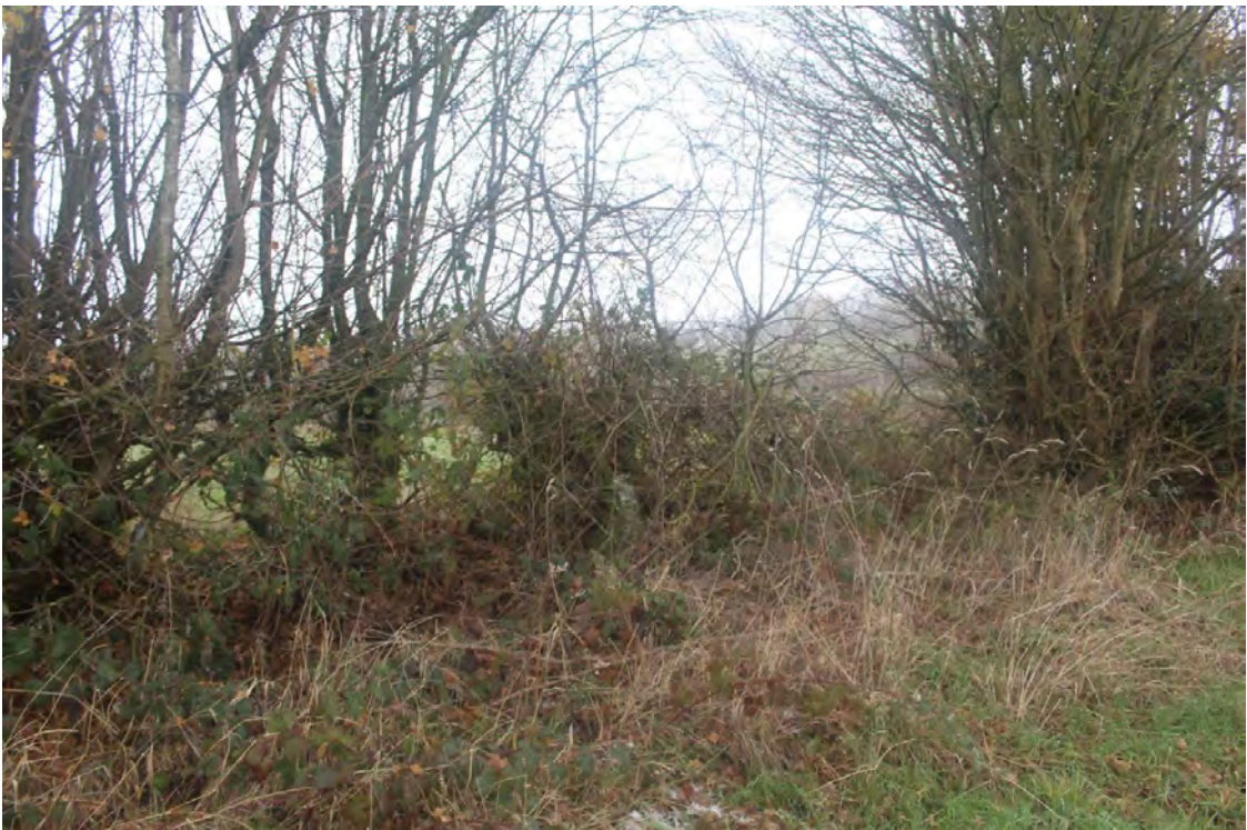
Image EDP A1.15: Close-up of the field boundary separating Fields 8 and 9 (from the east) and here illustrating that it is embanked and there is no associated ditch.
