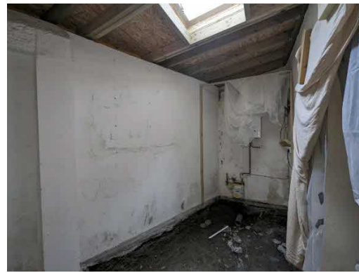
Photo 5. Showing the interior of the lean-to
