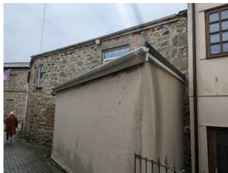
Photo 3. Showing the building from the north west and the lean-to
