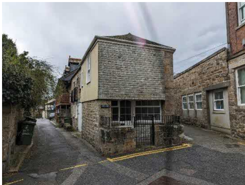
Photo 1. Showing the building from the east
