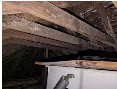
Photo 6. Showing the roof void over the eastern part of the building
