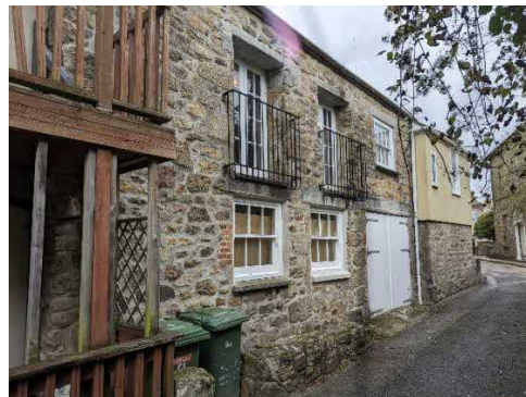
Photo 2. Showing the building from the south west
