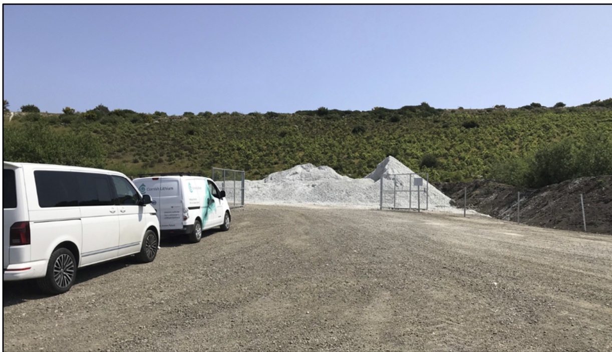
Figure 3.2: Newly Constructed Access Gate (Source: Site Visit, June 2023)
