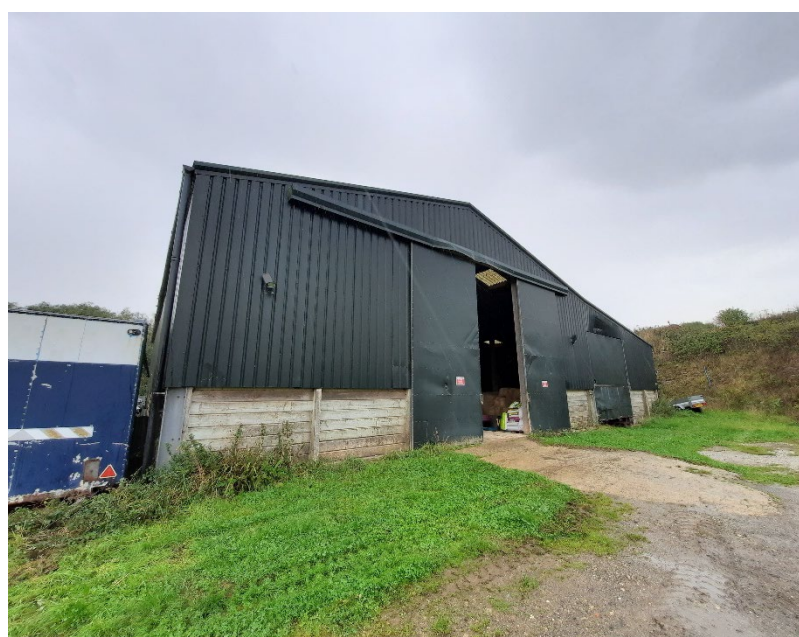
Figure 2: View of the western elevation of the barn.
