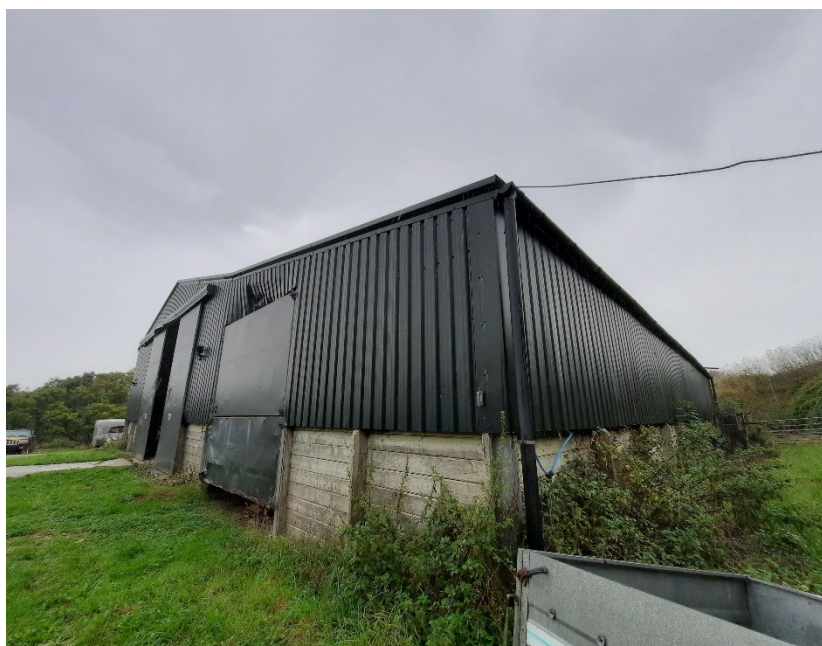
Figure 1: View of the south and west elevations of the barn.
