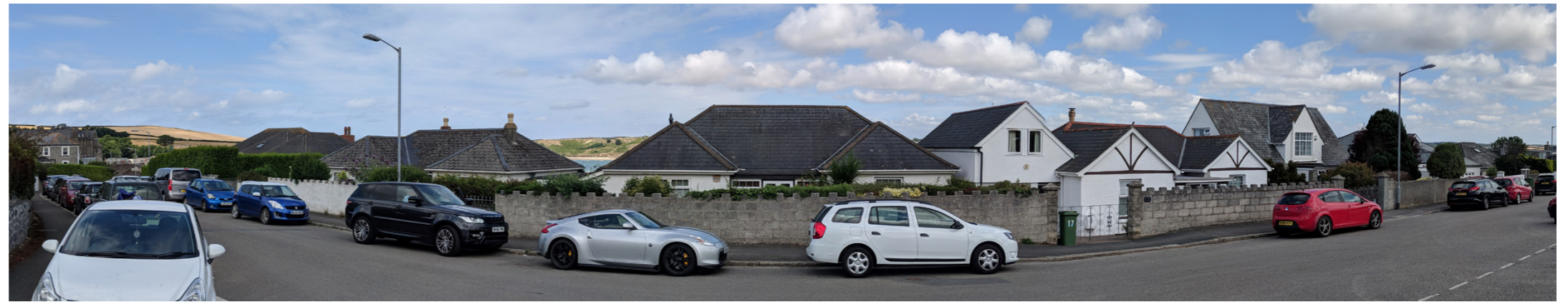
View from Egerton Road of 15 Treverbyn Road South West Elevation
