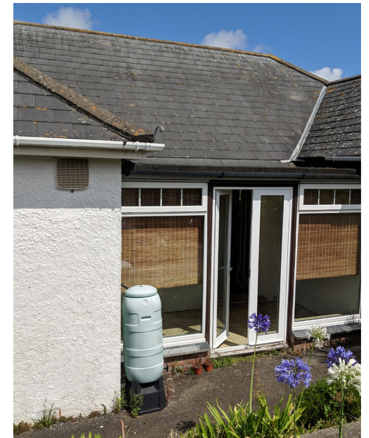
View of 15 Treverbyn Road Entrance
