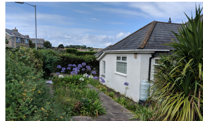
View of 15 Treverbyn Roadside Garden
