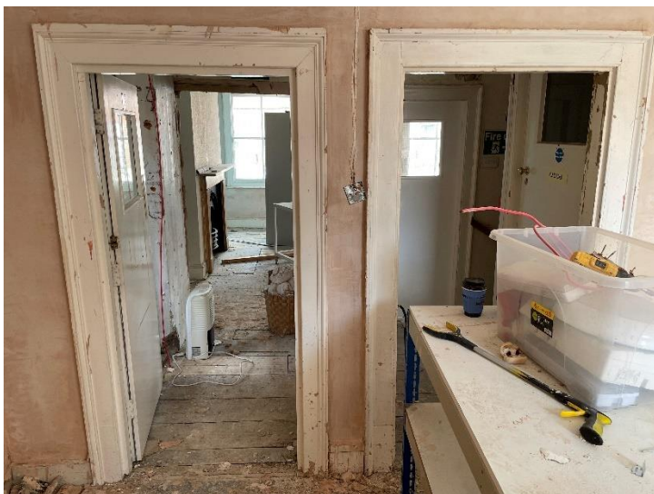
Plate 7: Double doorway within rear room.
