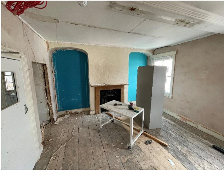
Plate 5: Front room, first floor; decorative mouldings on beam still present.
