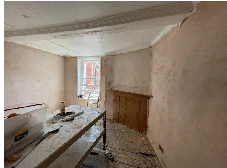
Plate 6: Rear room, first floor; decorative mouldings on beam still present.
