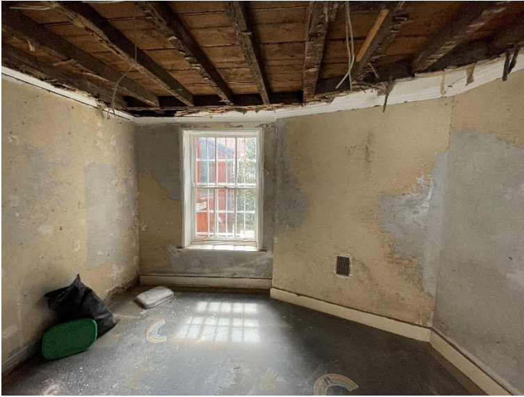
Plate 3: Rear room, ground floor.
