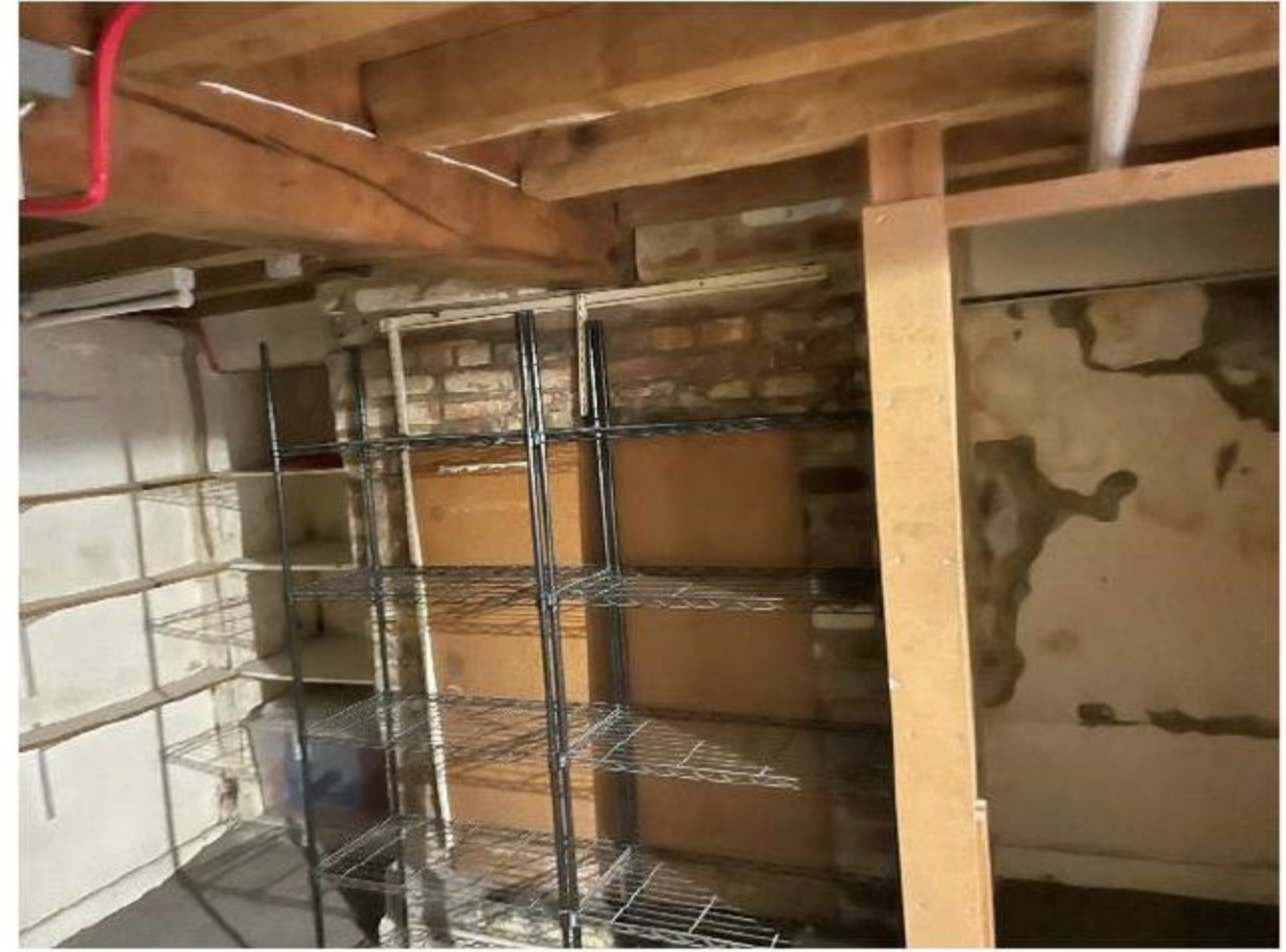
Figure 21 – Basement – modern joists supported on modern beam
