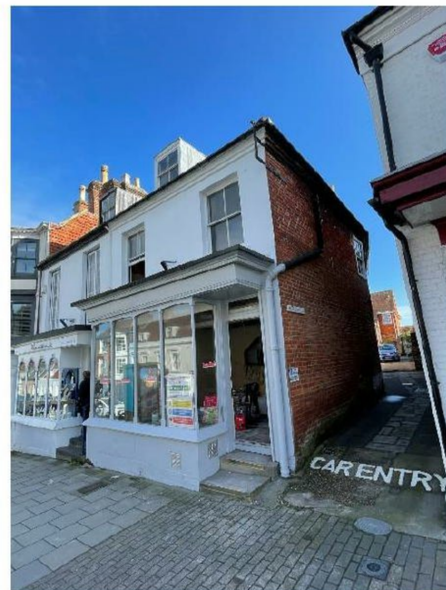
Figure 2 - Street view of 18 High Street
