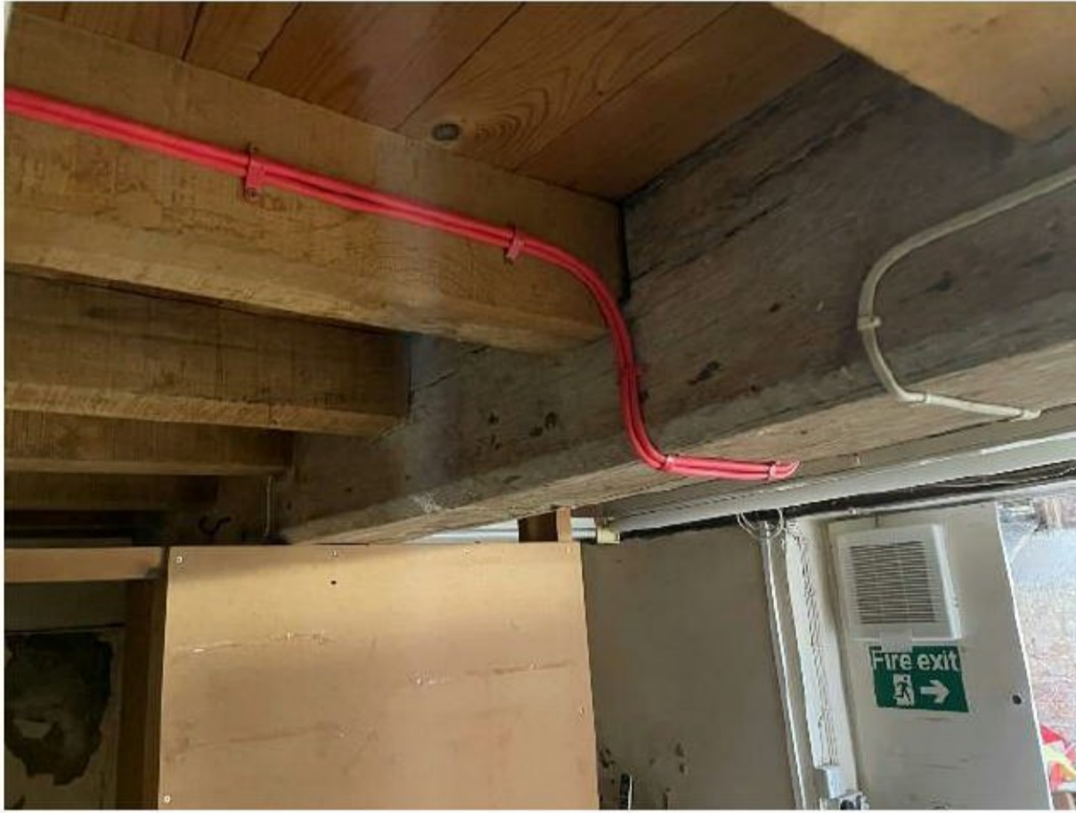
Figure 20 – Basement – modern joists supported on original beam
