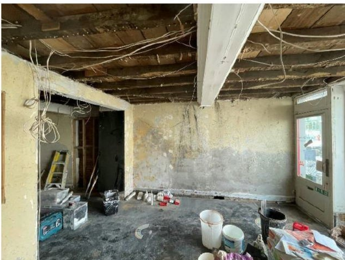
Figure 6 - View looking west of bays a and b
