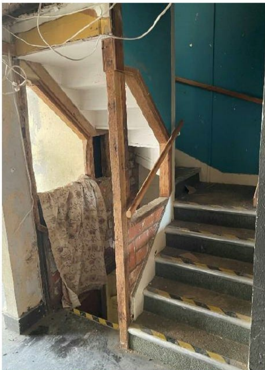
Figure 17 – Internal timber frame arrangements around staircase
