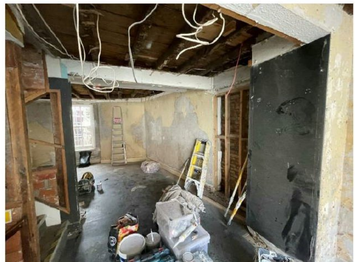
Figure 7 - View looking south of bays c and d
