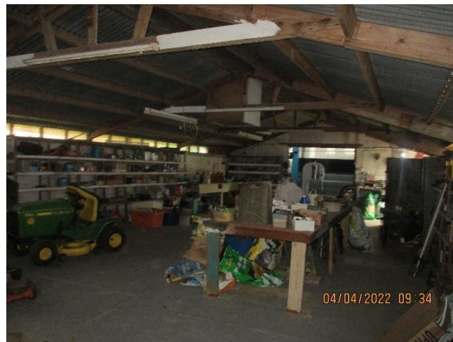
Photo 14: Interior of 'B1'.
