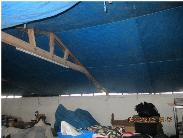
Photo 13: Interior of 'B1'.
