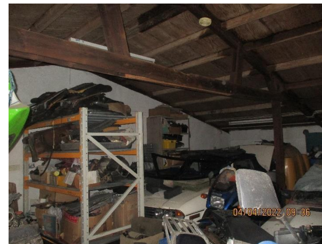
Photo 15: Interior of 'B3'.
