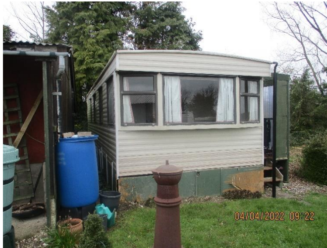
Photo 5: West elevation of 'B4'.
