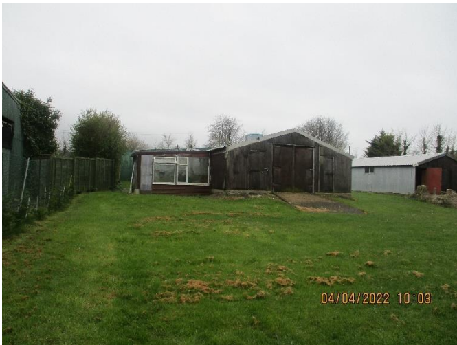
Photo 4: North elevation of 'B1'.
