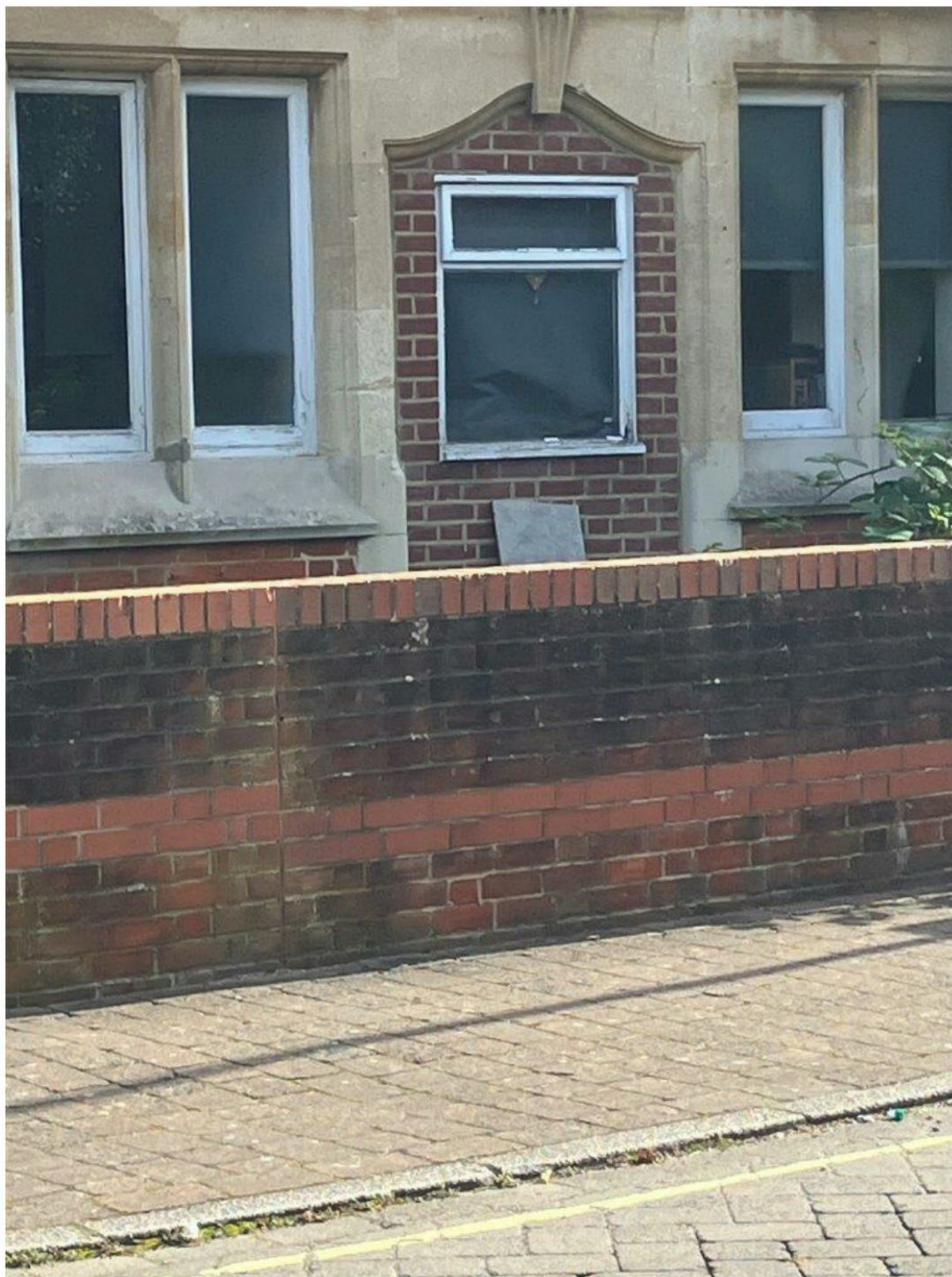
Plate 5 – Murrays Hotel – southwest elevation - non-original timber window installed as part of the conversion of the hotel into residential accommodation
