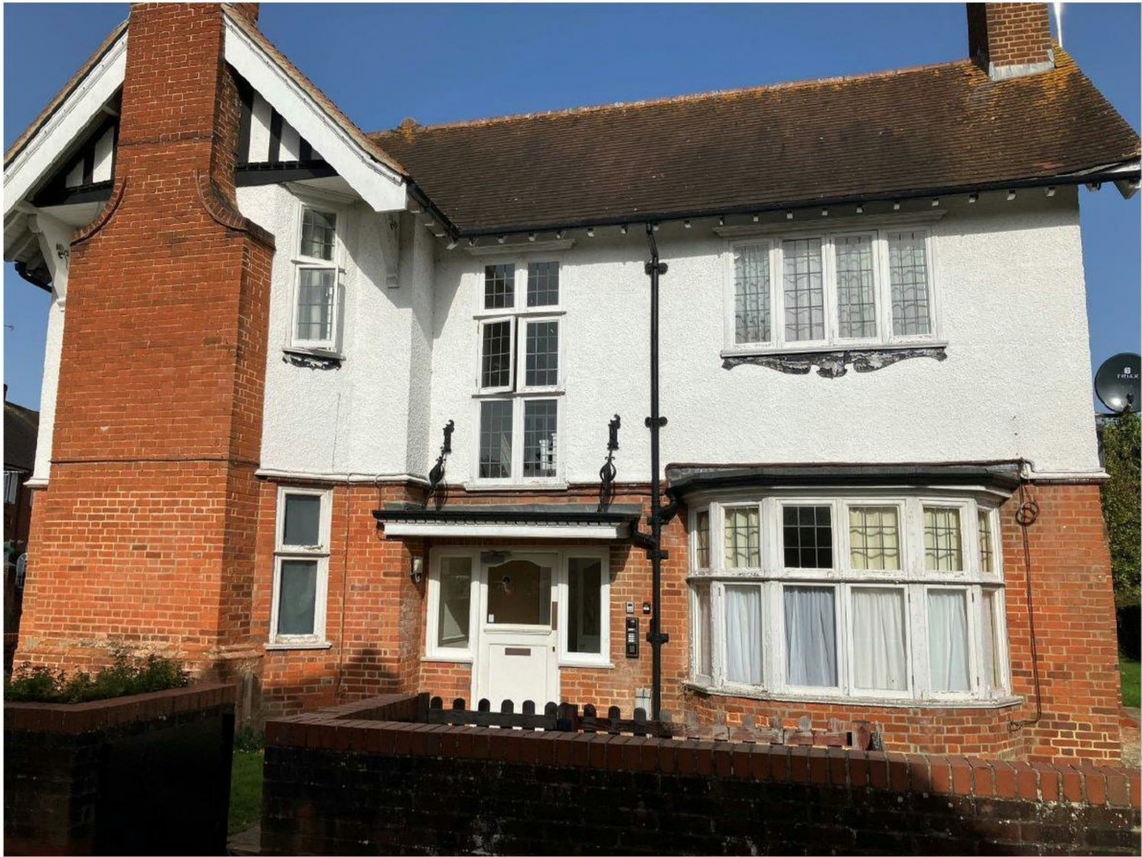
Plate 4 – Murrays Hotel – southeast elevation
