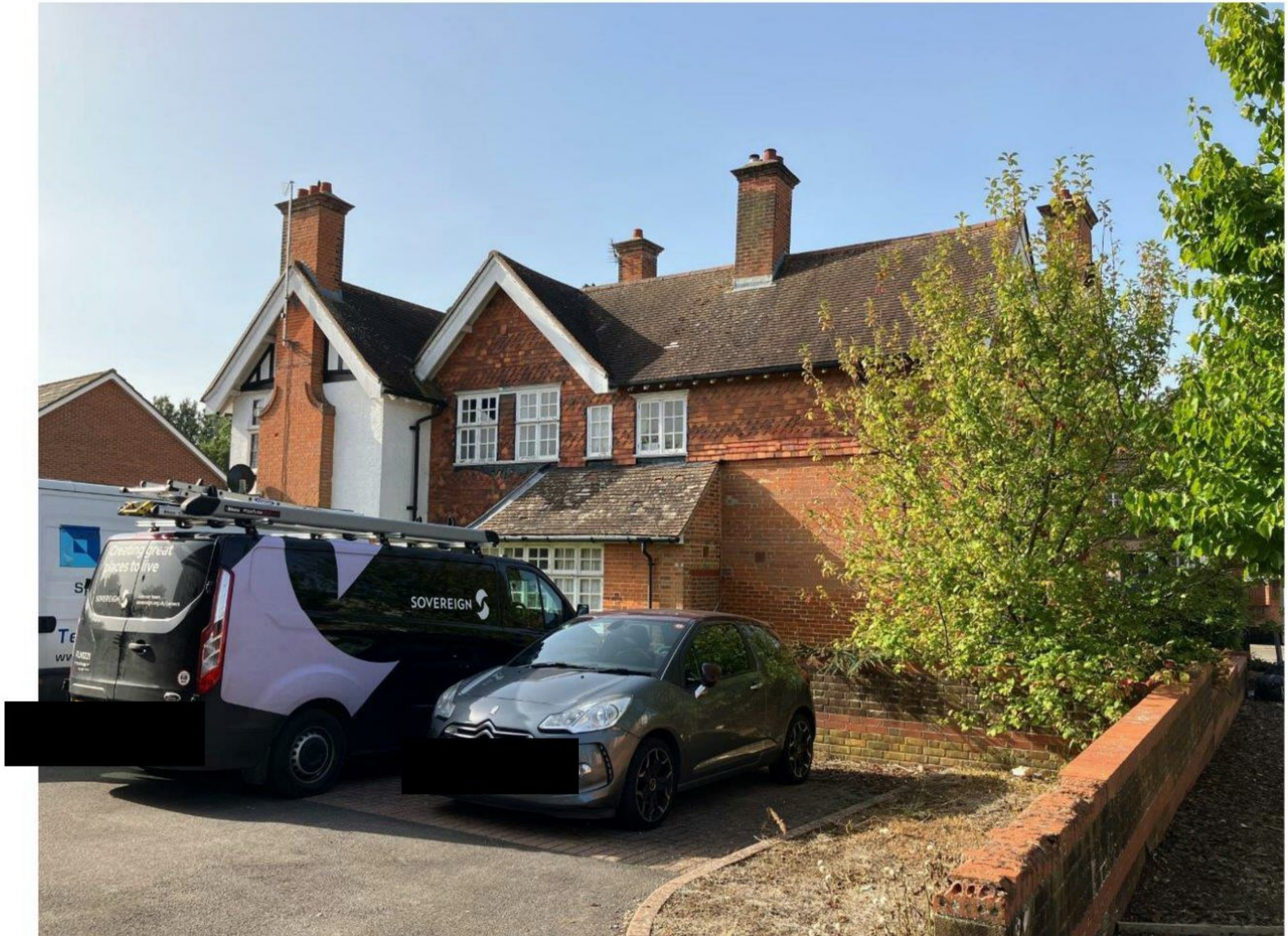
Plate 2: Murrays Hotel – northeast elevation.
