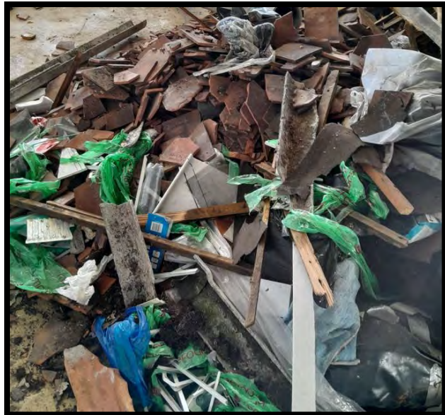
Photo 11 – Mixed waste with ACM
