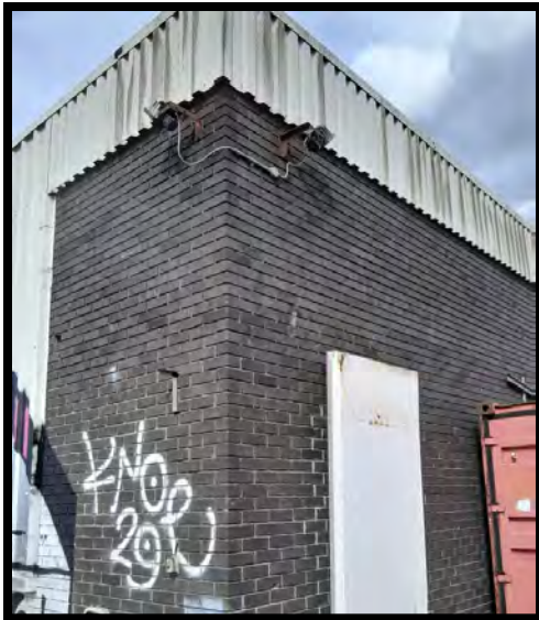
Photo 7 – Building Fabric Brick
