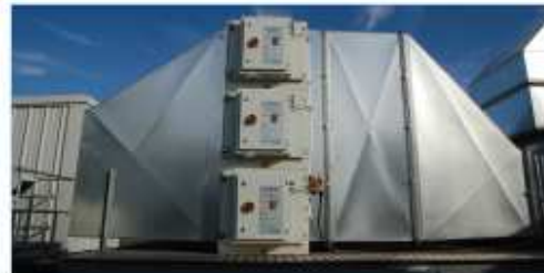
3 ESP Units Stacked in modular formation
