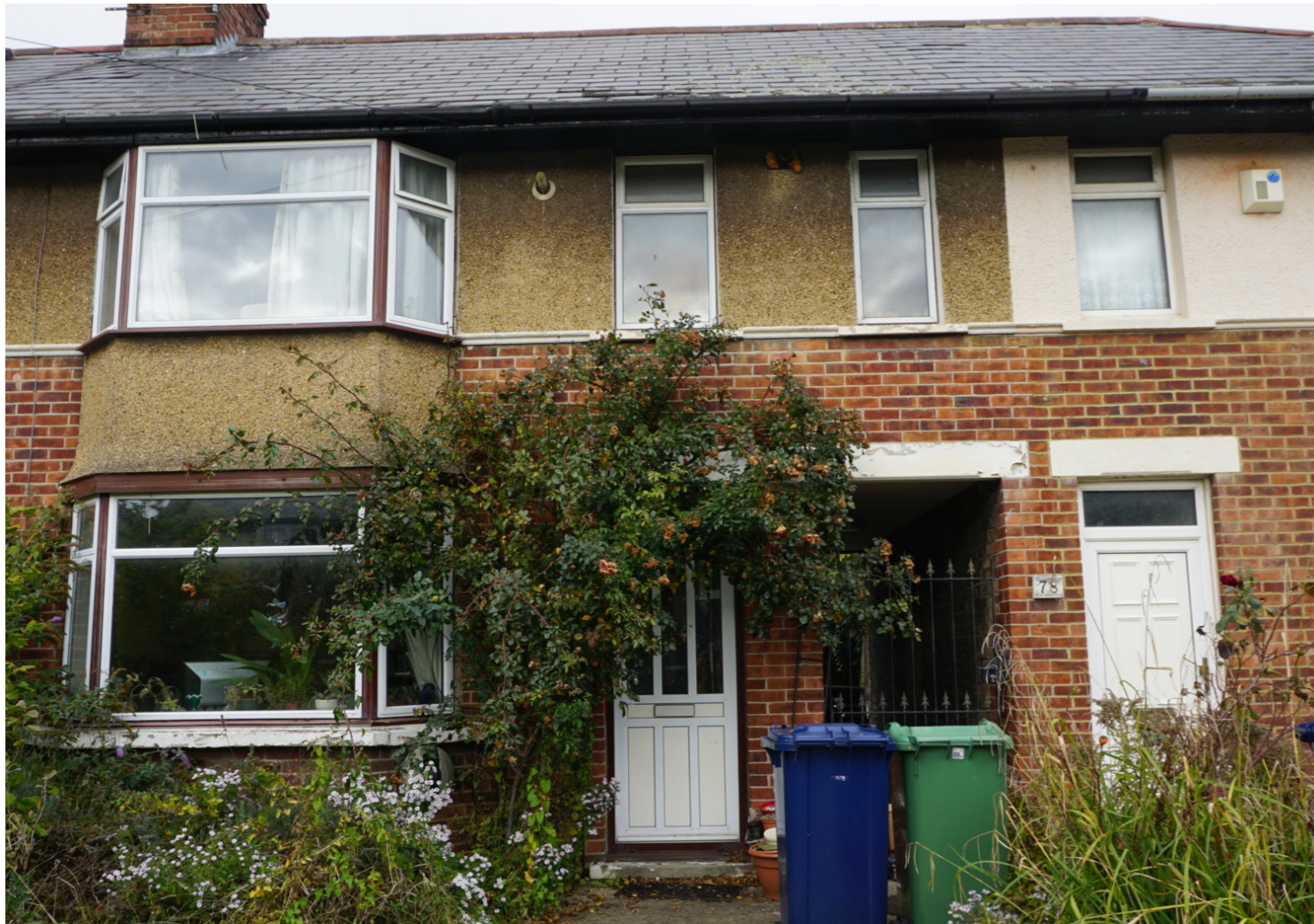
Above Front elevation image. Photo taken October 2022.
