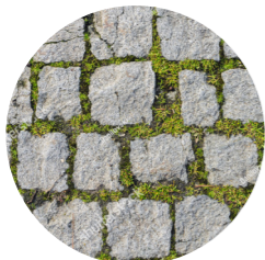
4 Permeable paving Permeable paving front driveway
