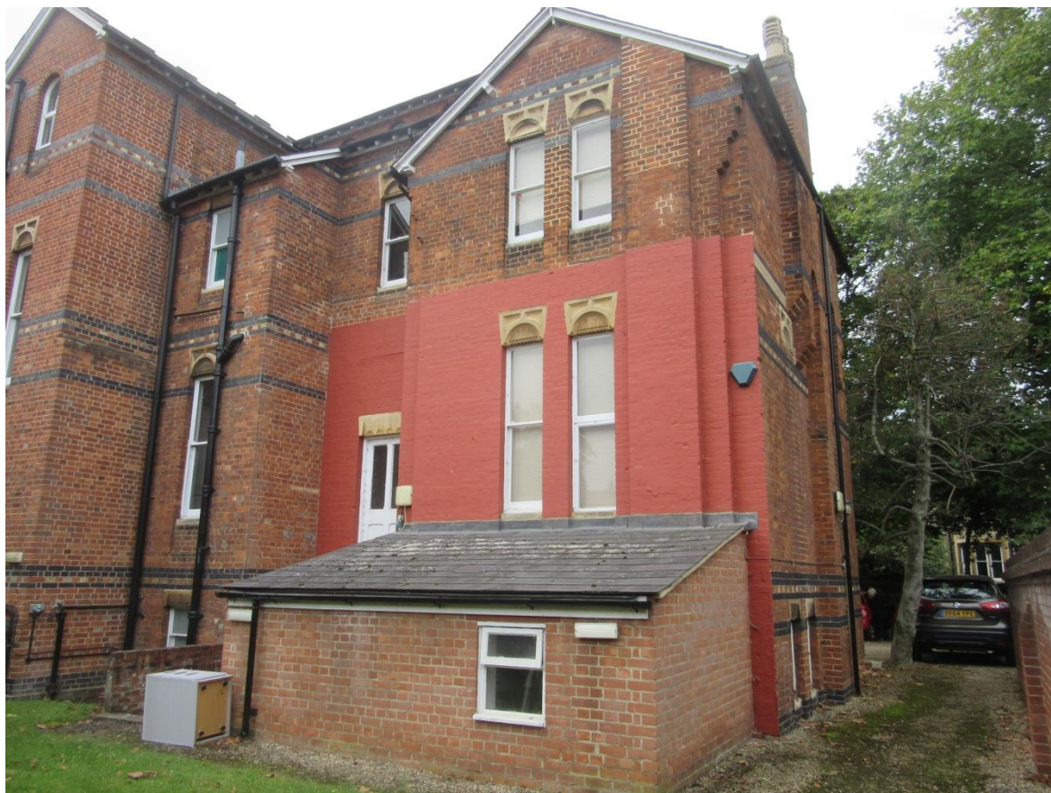
Figure 9: The unlisted No. 58 which encloses the subject site on the west side.
