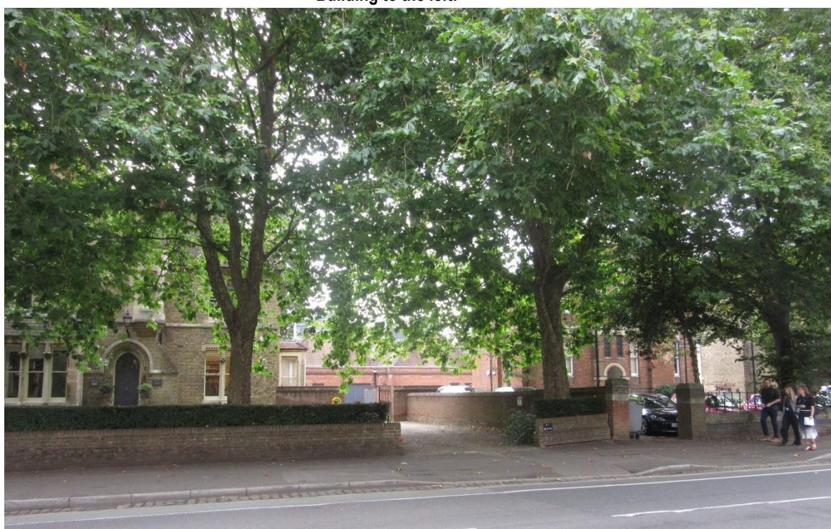
Figure 8: The Grade II listed No. 60 (left) and No. 58 (right) with the Balfour building in the gap; the forecourts are separated by an original boundary wall.
