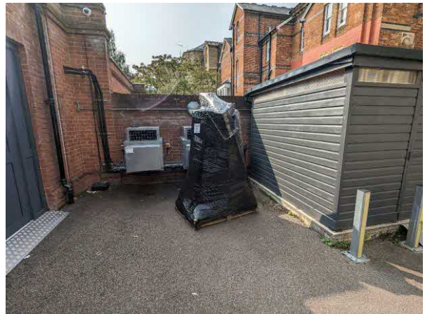
Photograph 4. The site, viewed from beyond the northern brick wall.
