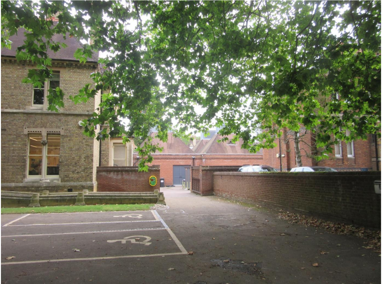
Figure 3a: View 02 as existing looking south-east from the east side of Banbury Road.
