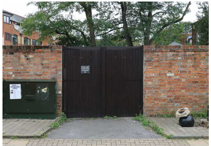
Fig. 6 - Solid gate opposite to the site
