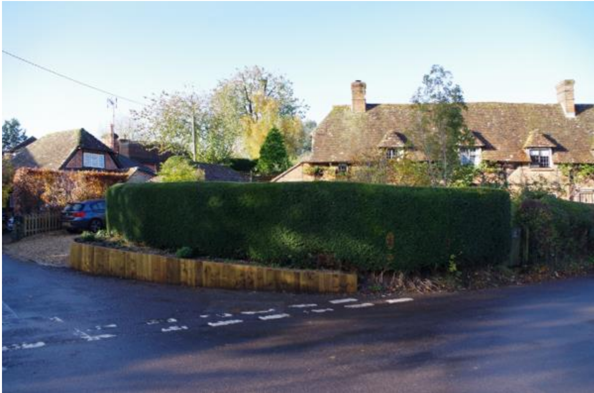
Photos of new retaining structure and associated planting.
