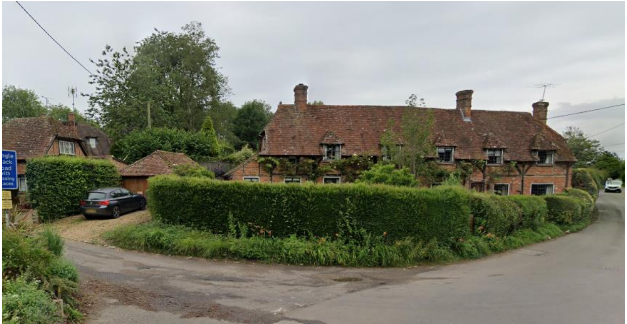
Street view - Corner Cottage showing the garden 'spillage' into Copse Lane prior to installation of the new retaining structure
