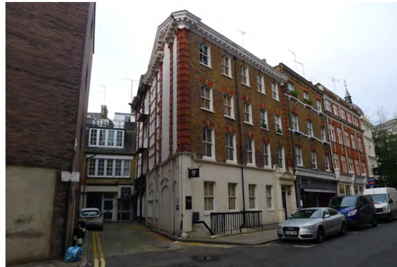
Mews buildings, Wells Street
