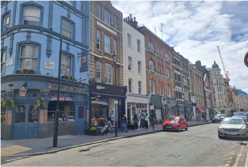
The range of commercial and residential buildings on Great Titchfield Street
