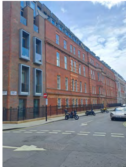
Historic facade of former hospital incorporated into new residential development, Nassau Street
