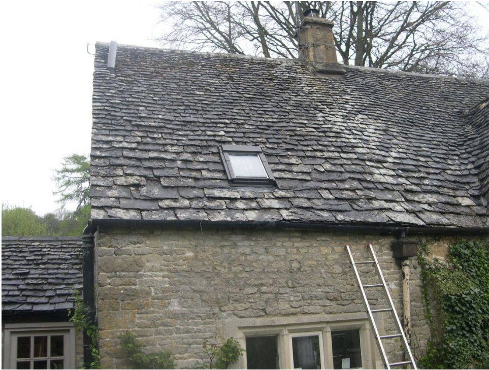
V. Roof window bedroom 2
