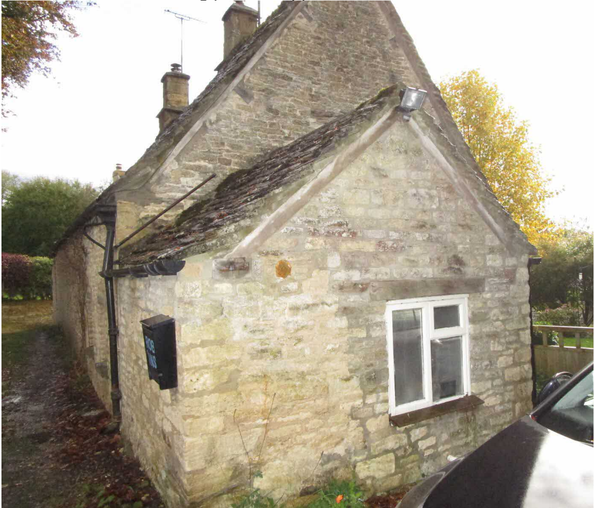
Figure 1 - The north western (side) & north-east (rear) elevations of the Cottage
