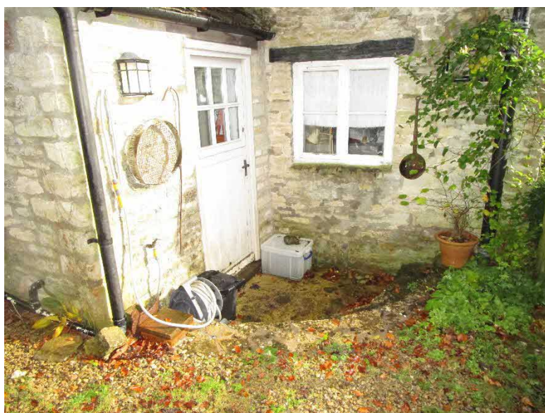
Figure 5– The hard standing by the existing cottage extension
