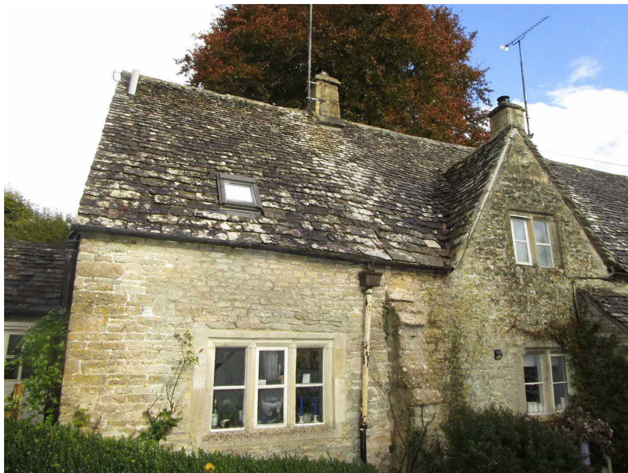
Figure 3 – The front (south west) elevation of the cottage
