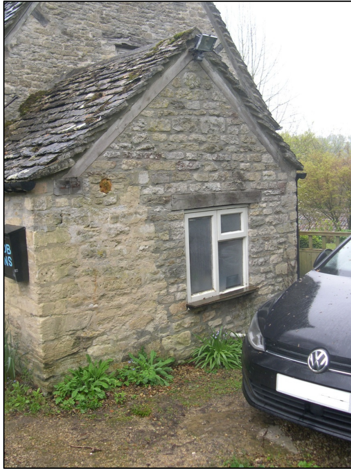
Photograph 2: Side (North-West) elevation, showing single-storey Kitchen extension ( to be demolished )
