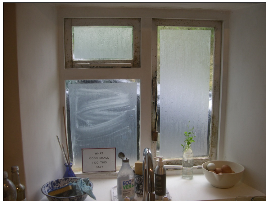
Photograph 5: Internal view of existing Kitchen window, to Side (North-West) elevation
