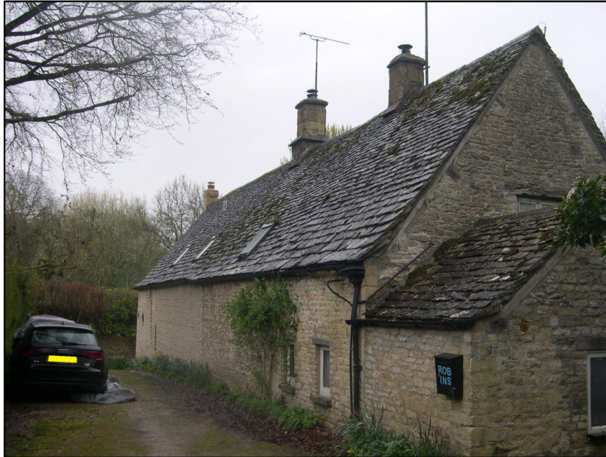
Photograph 1: Rear (North-East) elevation – existing single-storey Kitchen extension ( to be demolished ) shown
