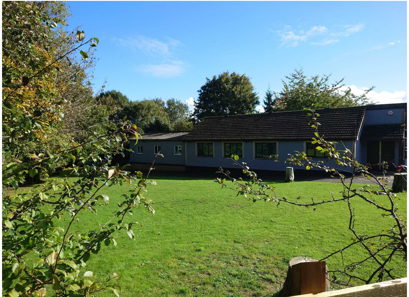
4. View from Public Highway
