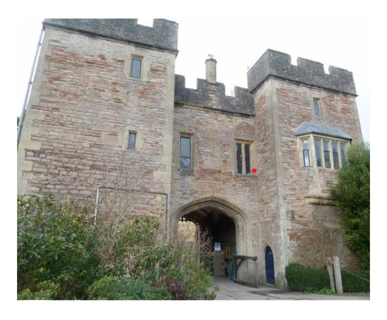
Cable entrance point into building. Through stone window frame 5 inches thick.
