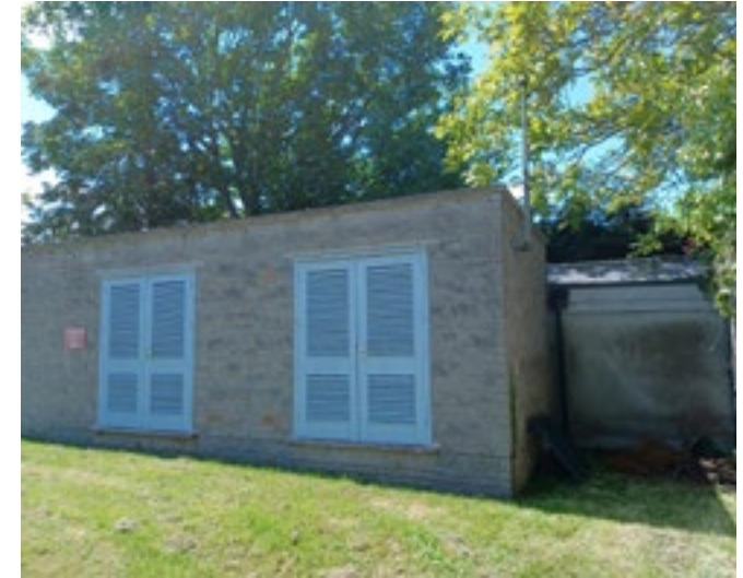
Gas Governor Building
