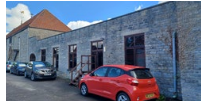
Link building – rear
