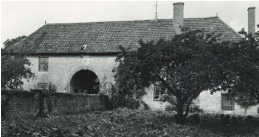
Barn in 1949, showing windows and doors prior to later alterations
