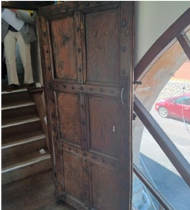
Barn interior - upper floor door
