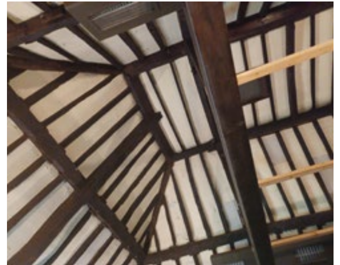
Barn upper floor - ceiling
