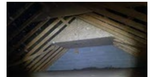
HOT BOX AT PITCH APEX
