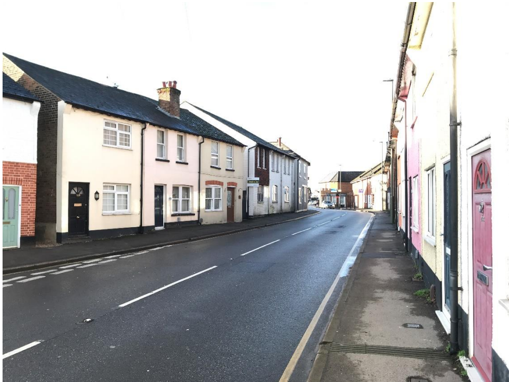
Plate 8: Typical view west on High Street looking toward 152 High Street.
