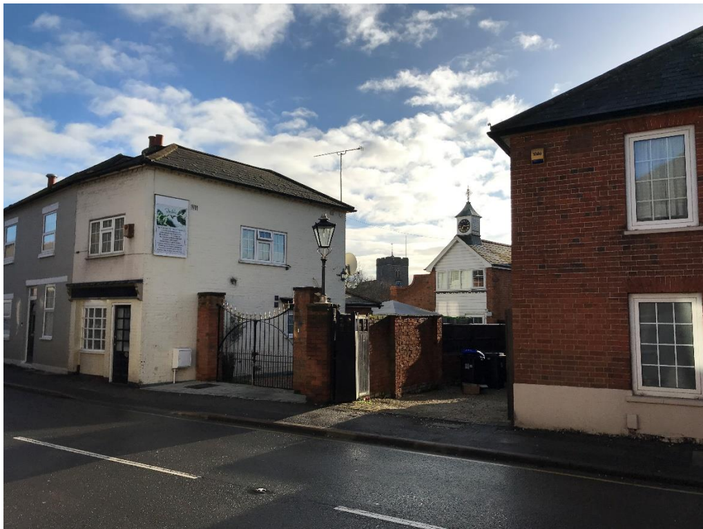
Plate 5: Typical view to St Peter's Church from High Street.
